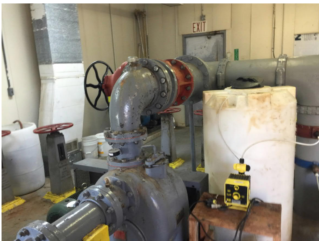
Figure 32: Phosphate Treatment Train - Intermediate Pump Station Piping
