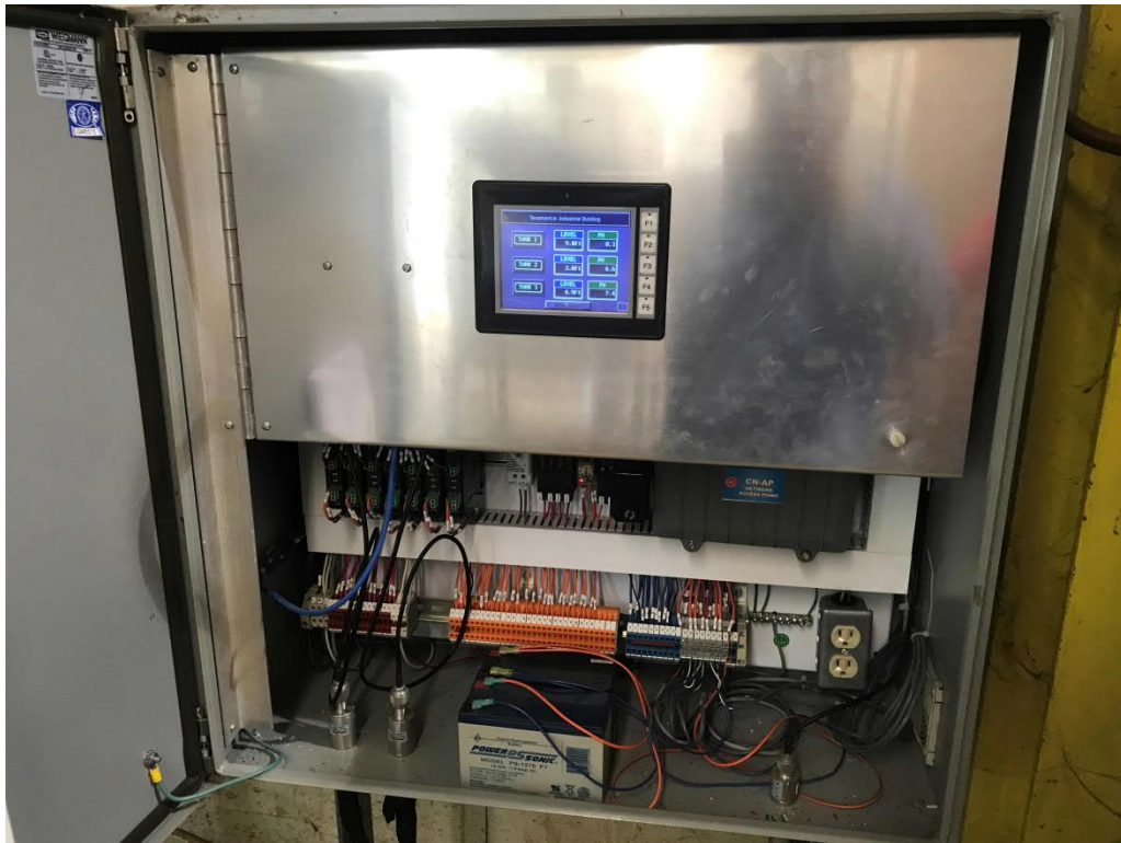
Figure 17: SCADA Control Panel
