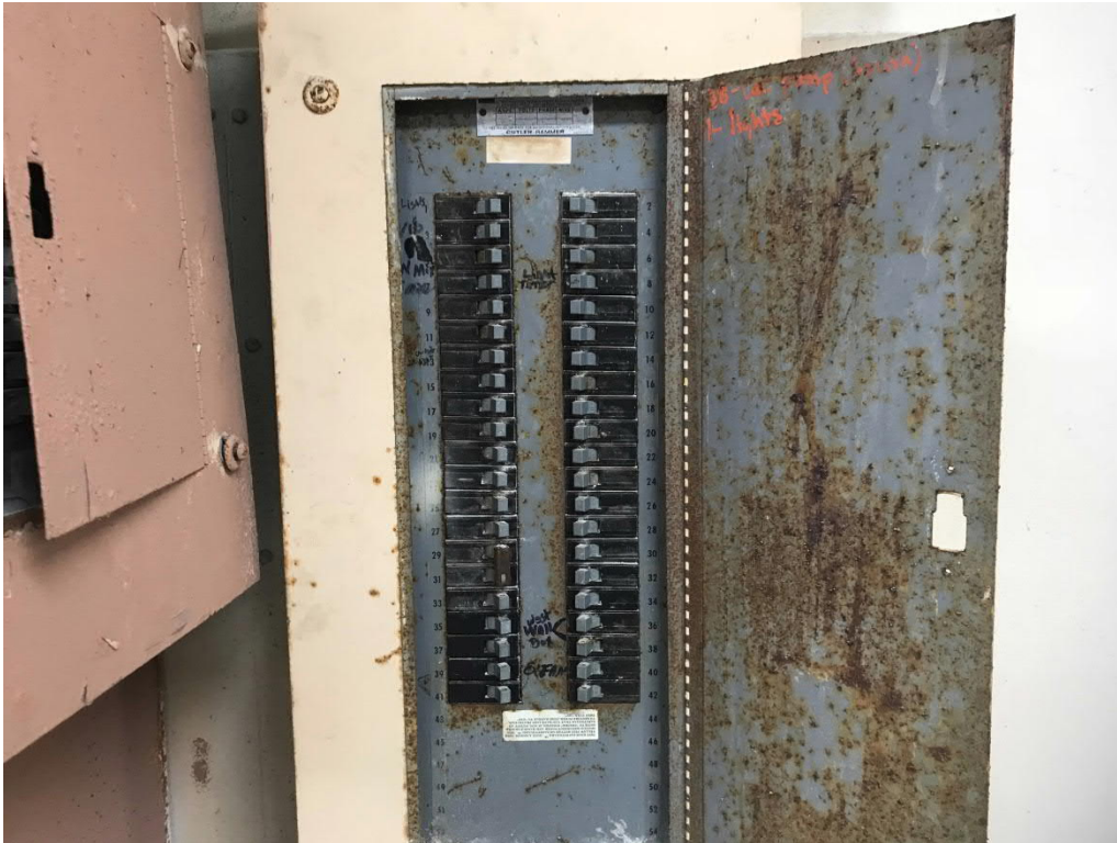
Figure 3: Chrome Building 480V panelboard with extensive corrosion
