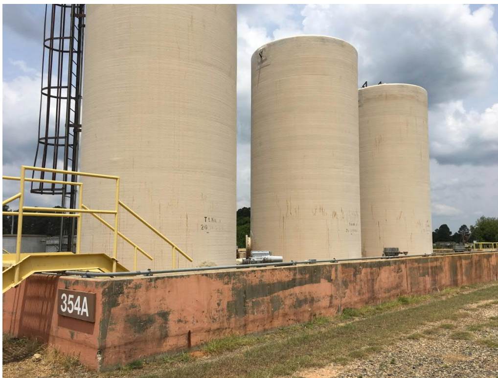
Figure 3: Chrome Treatment Train - Equalization Tanks
