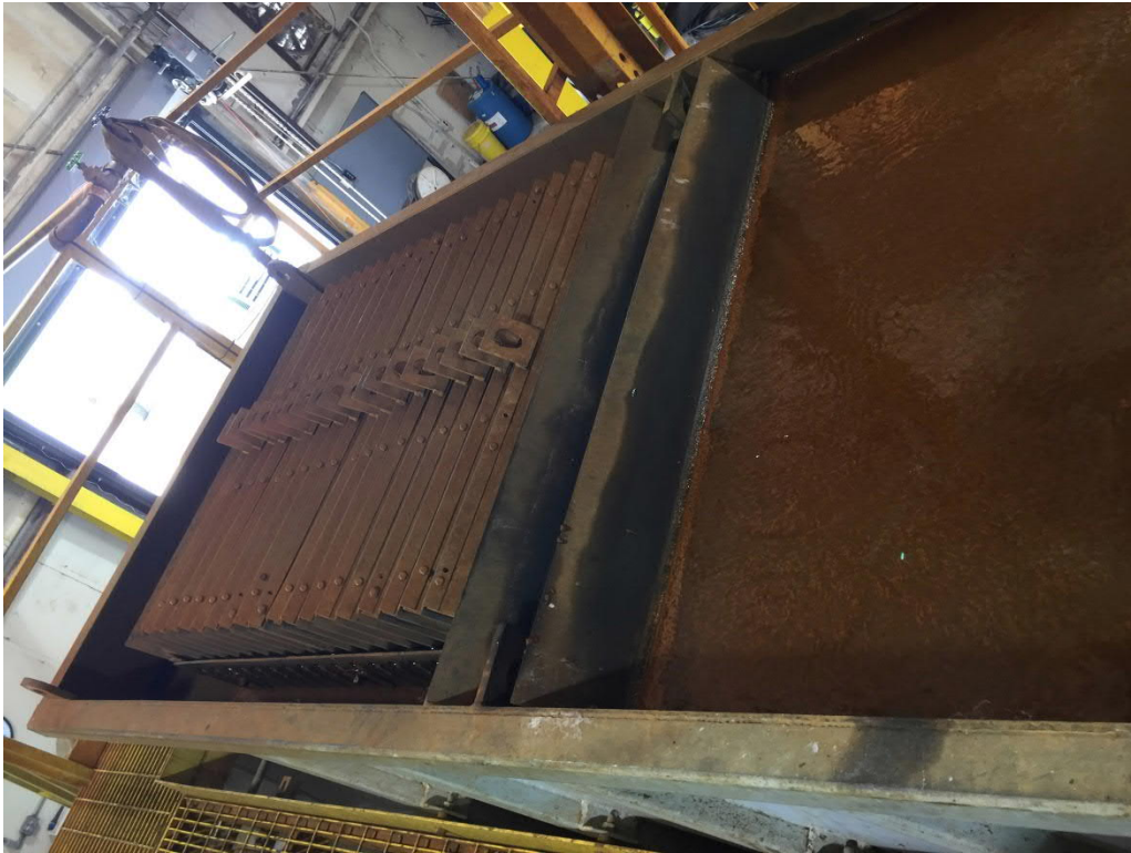
Figure 9: Chrome Treatment Train – Top of Inclined-Plate Clarifier
