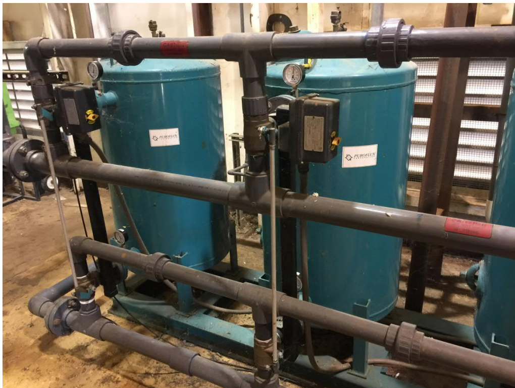
Figure 13: Chrome Treatment Train - Filters
