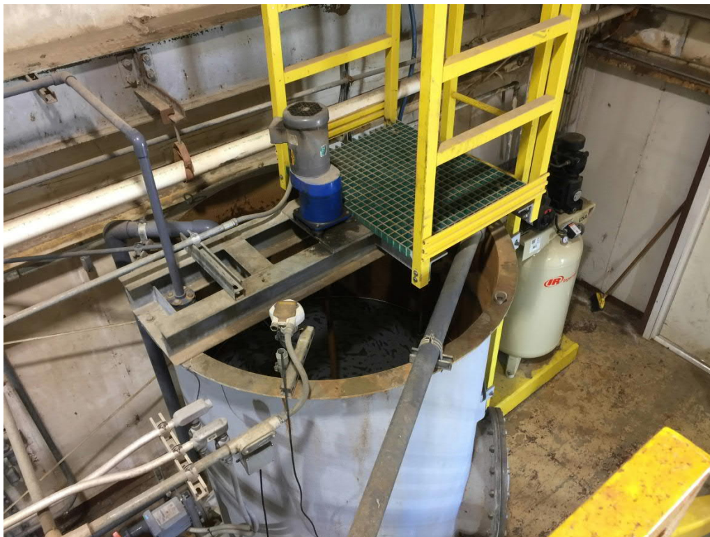
Figure 11: Chrome Treatment Train – Top of pH Adjust Tank
