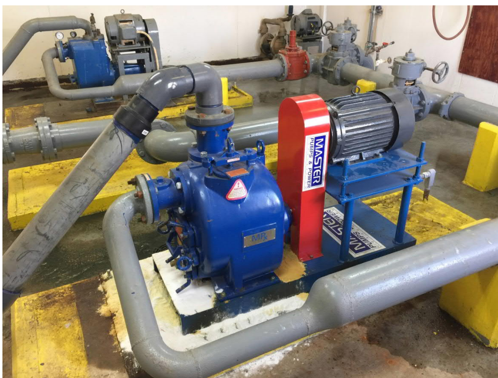
Figure 54: Phosphate Treatment Train – Sludge Pumps
