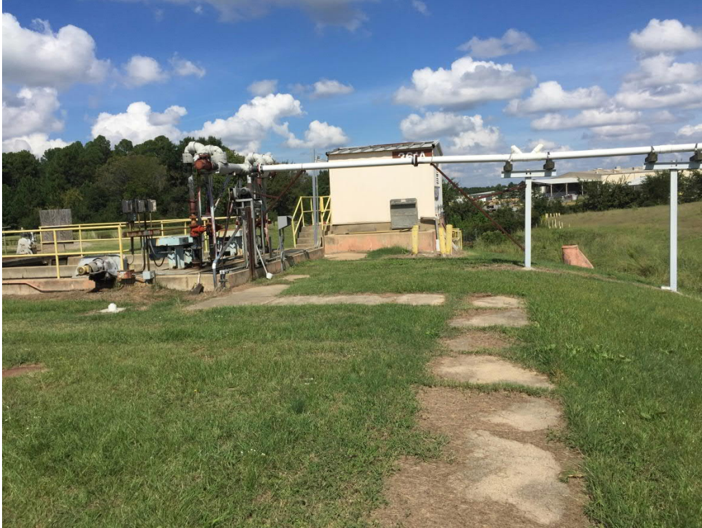
Figure 37: Phosphate Treatment Train - Grit Wash Pipe Line to Dewatering Beds
