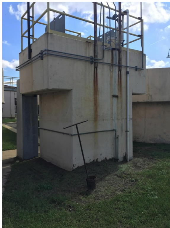
Figure 40: Phosphate Treatment Train - Polymer Mixing Tower
