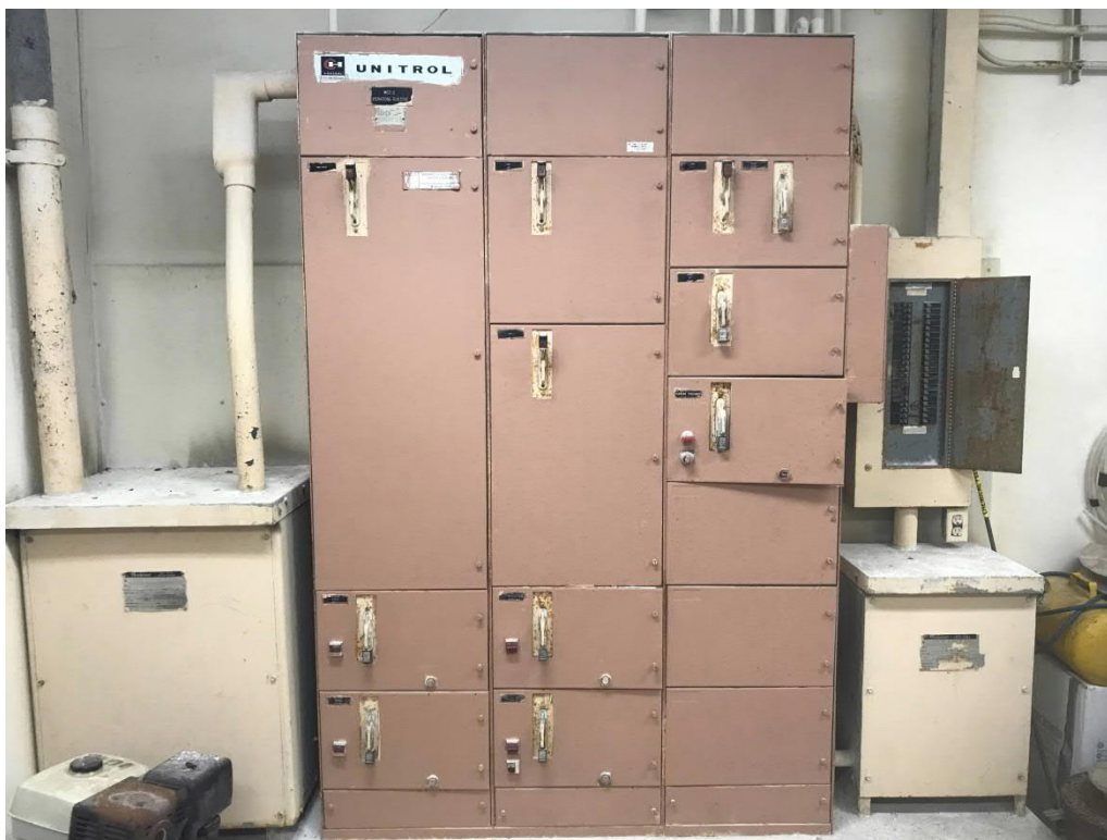
Figure1: Chrome Building 480V Motor Control Center
