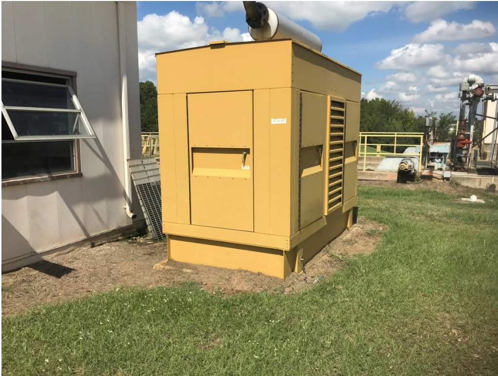
Figure 13: Phosphate Standby Generator
