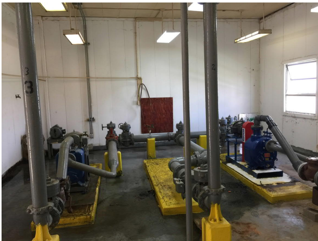
Figure 53: Phosphate Treatment Train – Sludge Pumps
