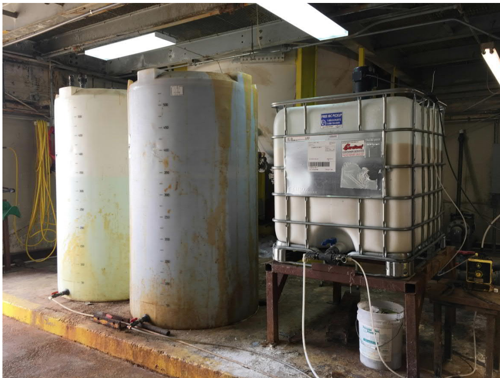
Figure 17: Chrome Treatment Train - Chemical Storage Tanks
