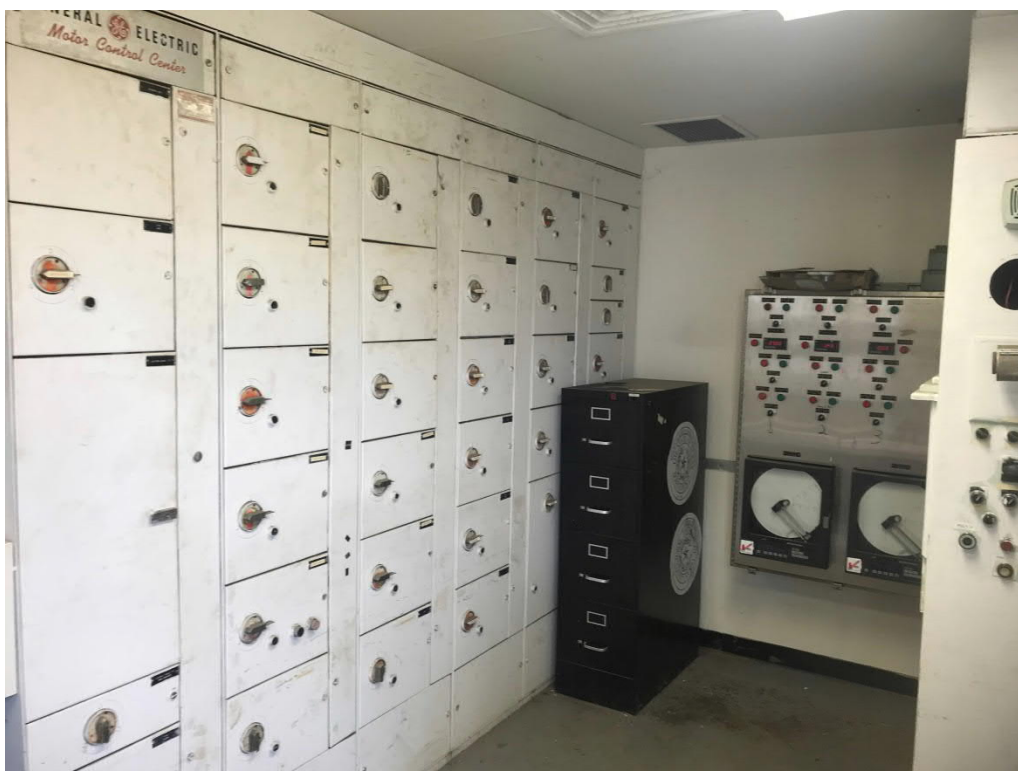
Figure 2: Chrome Building 208V Motor Control Center, insufficient working space per NEC requirements
