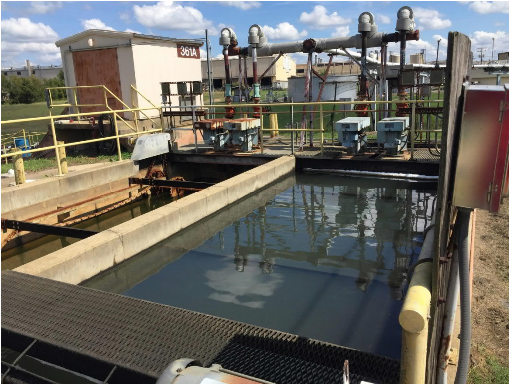
Figure 35: Phosphate Treatment Train - Oil-Water Separator
