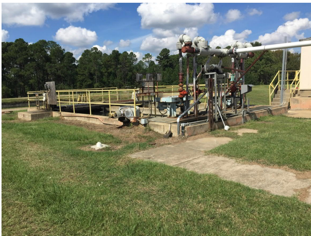
Figure 34: Phosphate Treatment Train - Oil-Water Separator
