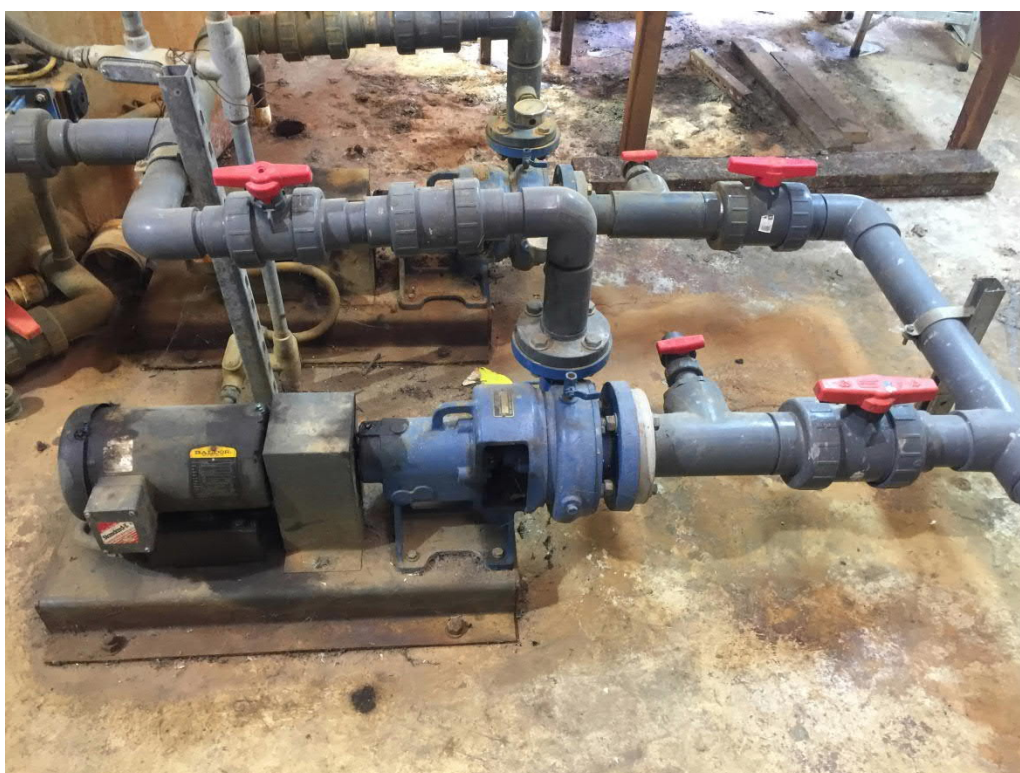
Figure 16: Chrome Treatment Train Tank Feed Pumps
