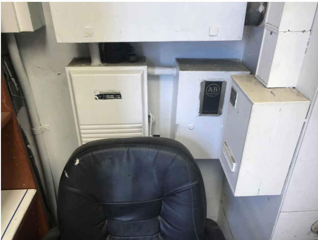
Figure 4: Electrical equipment in Chrome Building with insufficient working space per NEC requirements
