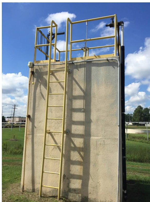
Figure 50: Phosphate Treatment Train - Clarifier Effluent Tower
