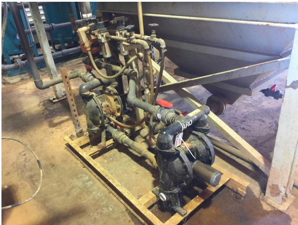
Figure 15: Chrome Treatment Train Diaphragm Recycle Pumps
