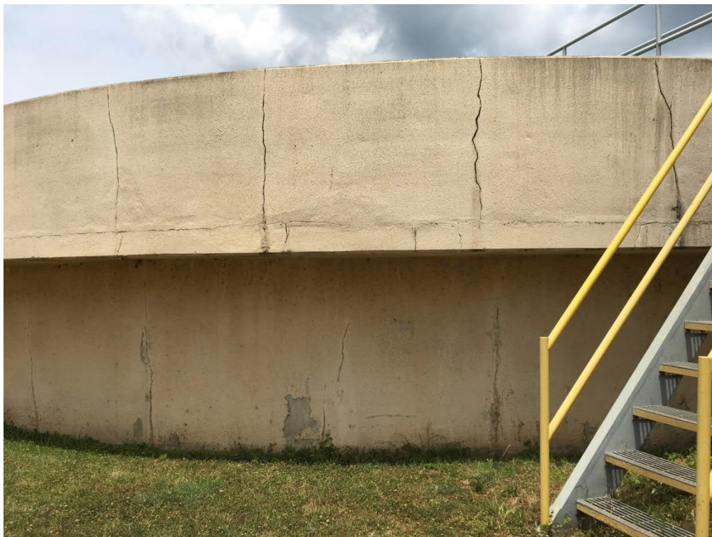
Figure 43: Phosphate Treatment Train - Cracking in Clarifier Walls
