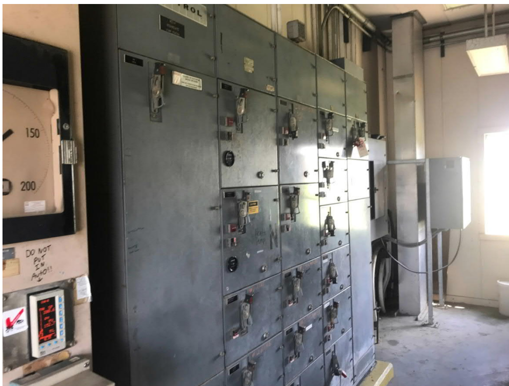
Figure 11: Phosphate 480V Motor Control Center
