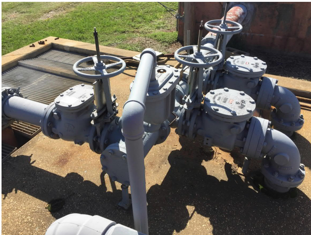
Figure1: Chrome Treatment Train - Lift Station
