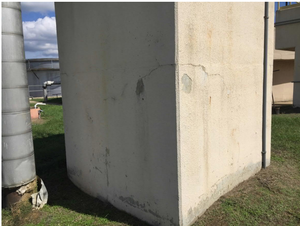
Figure 51: Phosphate Treatment Train - Crack in Clarifier Effluent Tower
