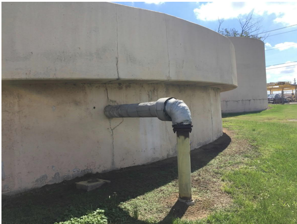
Figure 45: Phosphate Treatment Train - Cracking in Clarifier Walls
