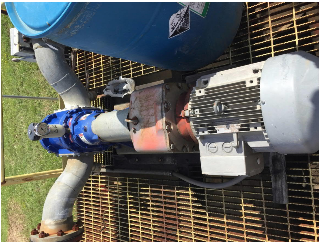
Figure 29: Phosphate Treatment Train - Influent Lift Station Spare Pump
