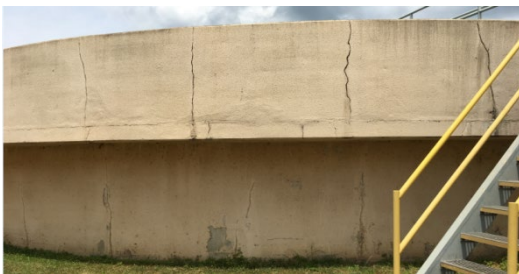
Figure 2: Secondary clarifier, noting cracks
