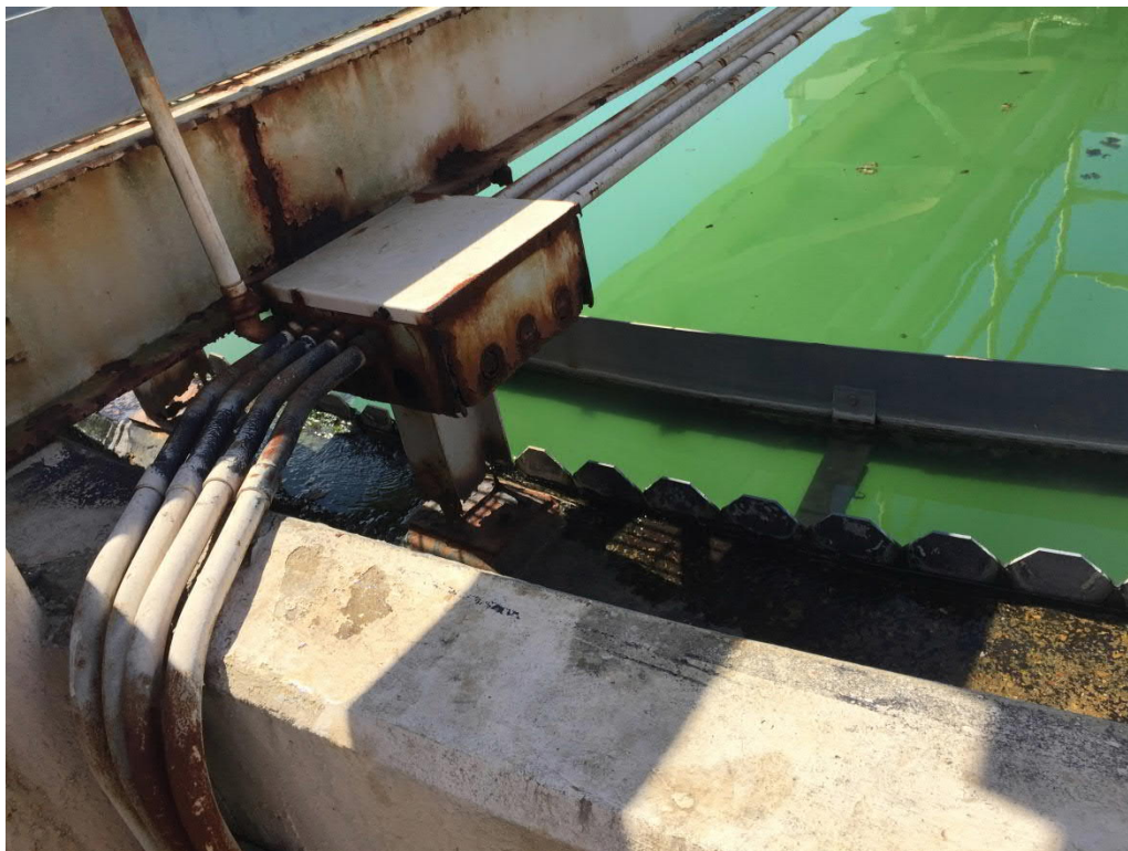
Figure 49: Phosphate Treatment Train - Extreme Corrosion in Clarifier
