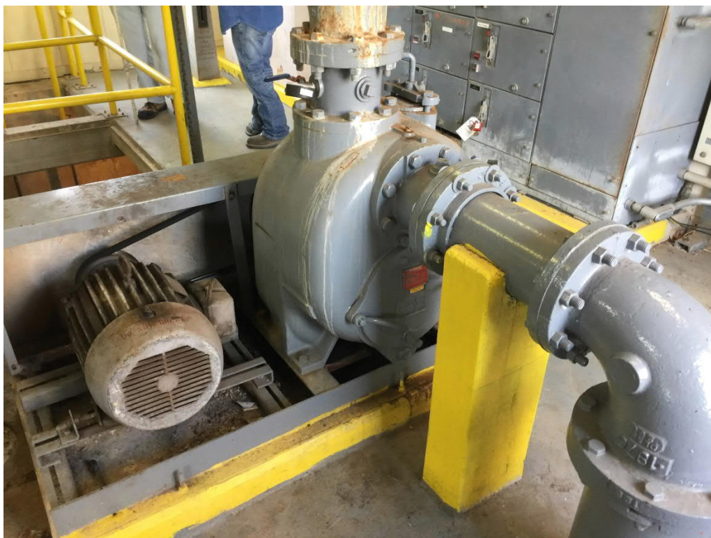
Figure 31: Phosphate Treatment Train - Intermediate Pump Station Pump
