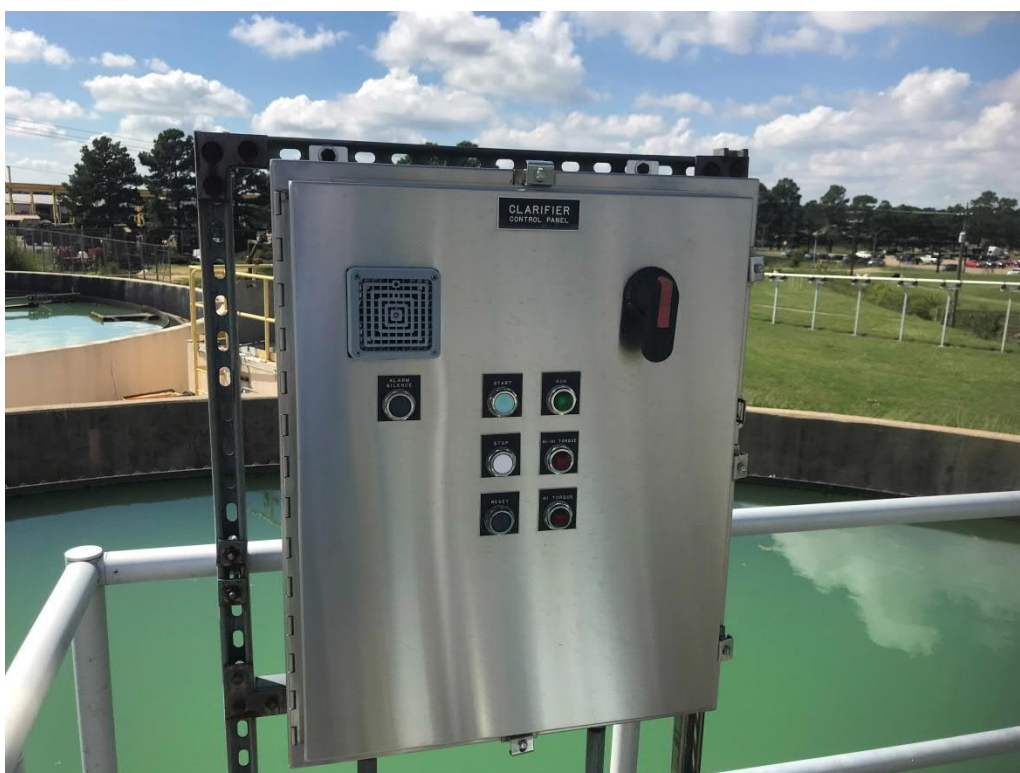
Figure 16: Rehabilitated Clarifier control panel
