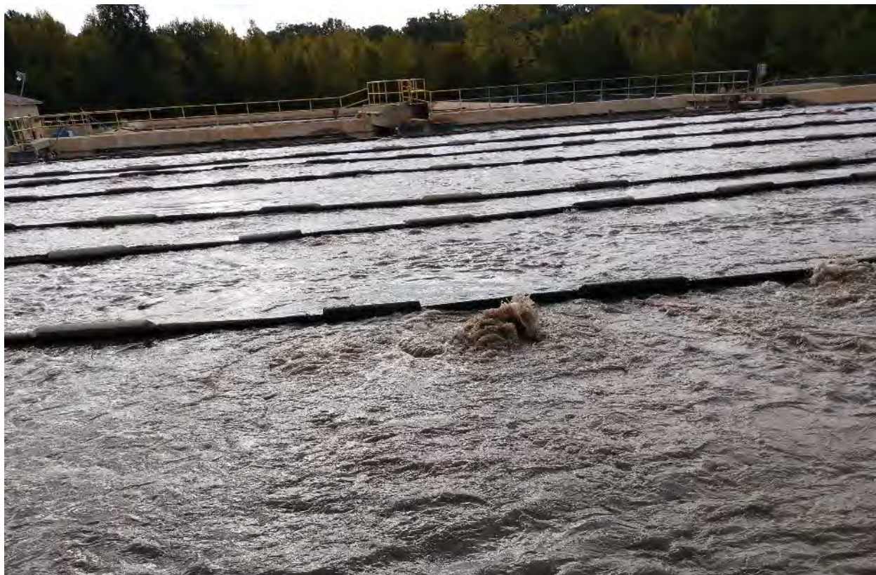
Figure 1.9: Aeration System, Diffusers range from little to no flow (far left) to blown pipe with direct flow (center) Surface of Aeration Basin should be relatively calm with evenly distributed flow.
