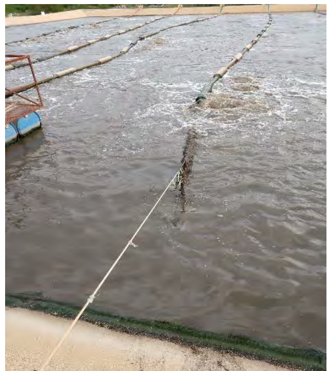
Figure 1.11: Blown Out Diffuser in Need of Repair.
