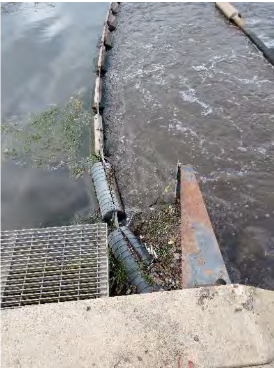
Figure 1.19: Surface Debris and Algae Build up In North Clarifier
