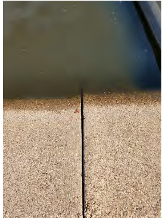
Figure 1.27: Joint Separation Along South end of Polishing Basin
