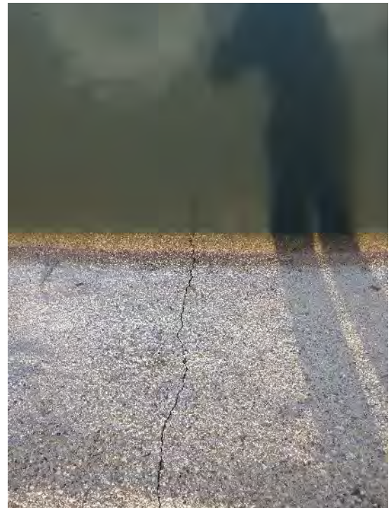
Figure 1.25: Cracking along Polishing Basin Apron
