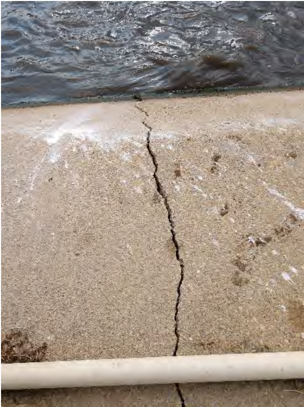
Figure 1.5: Significant Cracking on West Side of Basin
