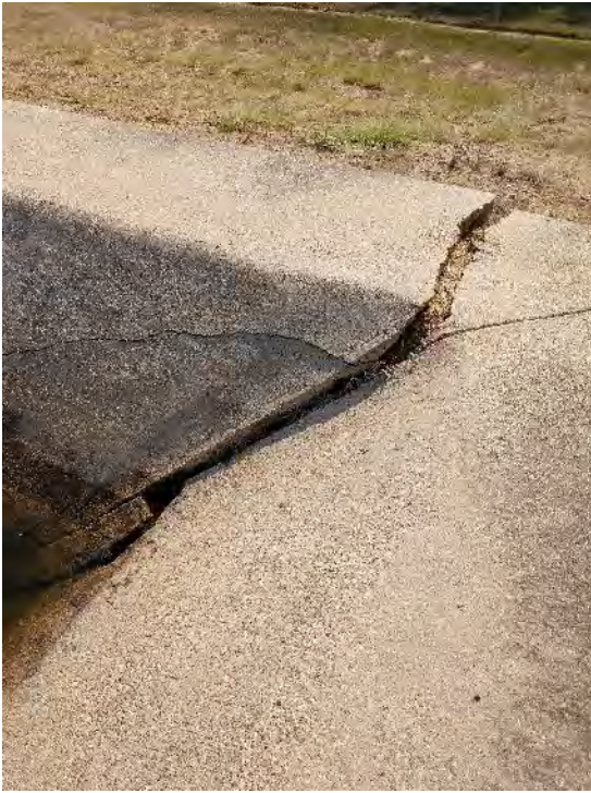
Figure 1.26: Significant Cracking and Separation at Southeast corner of Polishing Basin
