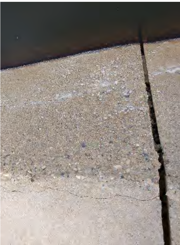
Figure 1.7: Significant Joint Separation and Cracking on East Side of Basin
