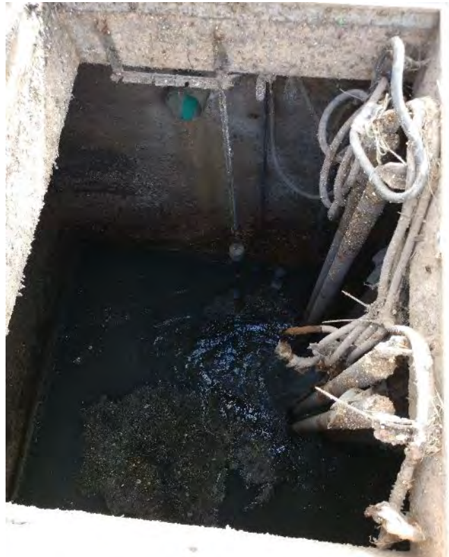
Figure 1.2: Wet Well and Lift Pumps
