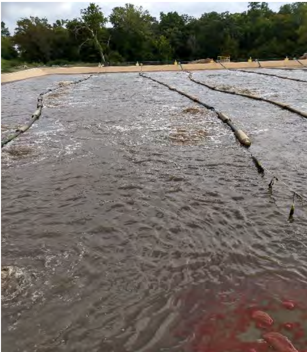
Figure 1.10: “Dead” Area in Basin due to Low Oxygen Flow Debris hanging from support cables throughout Pond
