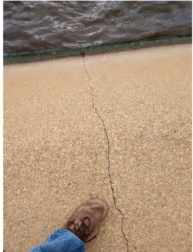
Figure 1.6: Cracking on South Side of Basin
