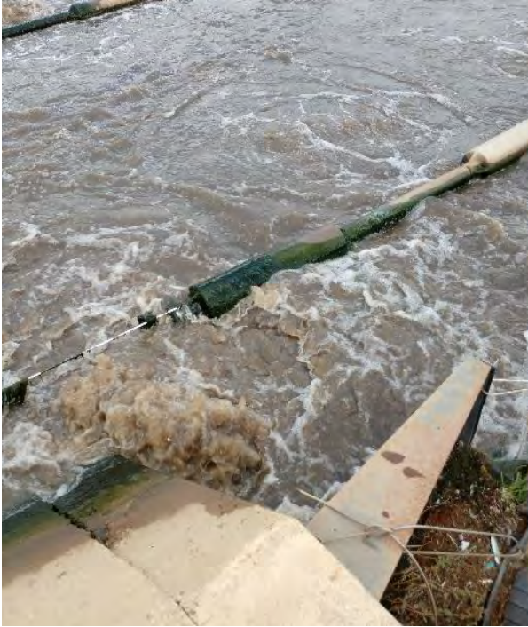
Figure 1.12: Blown Out Diffuser Adjacent to Large Joint Separation and Debris Pile on Surface of Basin
