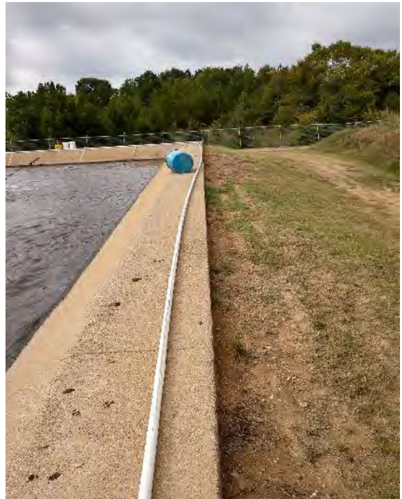
Figure 1.15: PVC Pipe Diffuser System, added to Decrease Dead Zones
