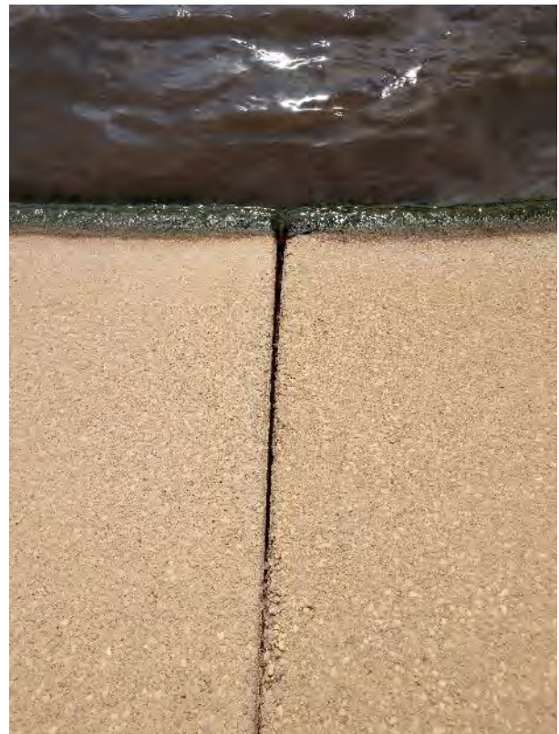
Figure 1.4: Concrete Joint Separation on West Side of Aeration Basin, Possible infiltration into surrounding soils
