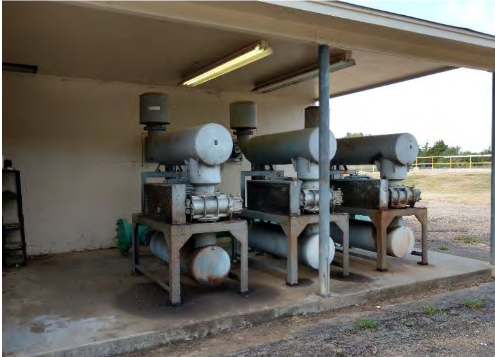
Figure 1.16: 3 Blowers Used to Maintain Aeration System. All three are currently being utilized to maintain basin.
