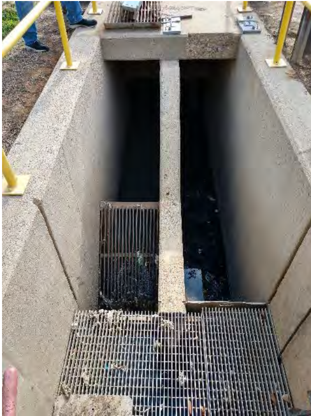
Figure 1.1: Manual Bar Screen & Entrance to Lift Station
