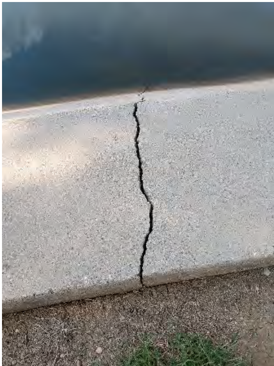
Figure 1.24: Significant Cracking north side of Polishing Basin
