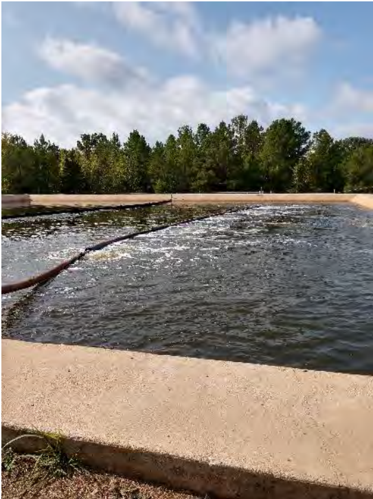
Figure 1.21: Polishing Pond and Biolac Aeration System
