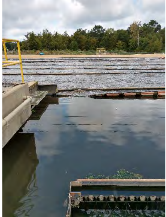
Figure 1.18: Breach in the North Clarifier Curtain Wall
