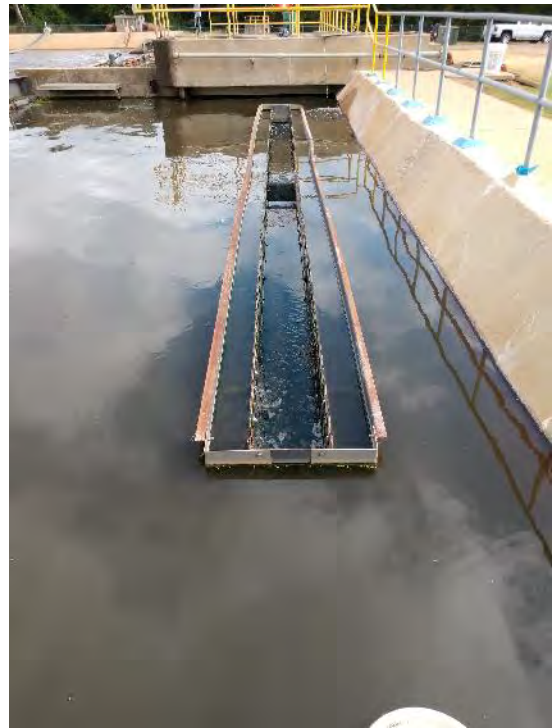
Figure 1.20: South Clarifier Weir Structure (Flocculation Rake inactive)
