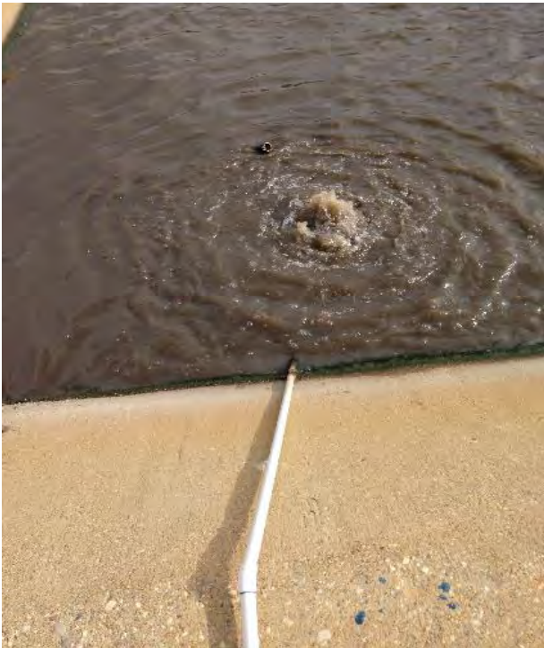
Figure 1.14: PVC Pipe added Diffuser System
