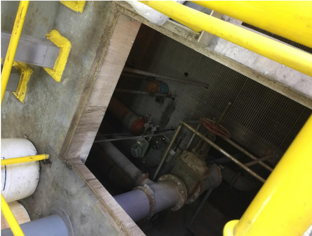
Figure 33: Phosphate Treatment Train - Intermediate Pump Station
