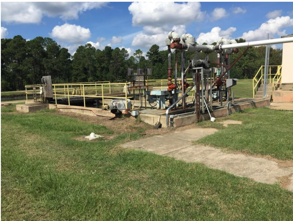
Figure 34: Phosphate Treatment Train - Oil-Water Separator
