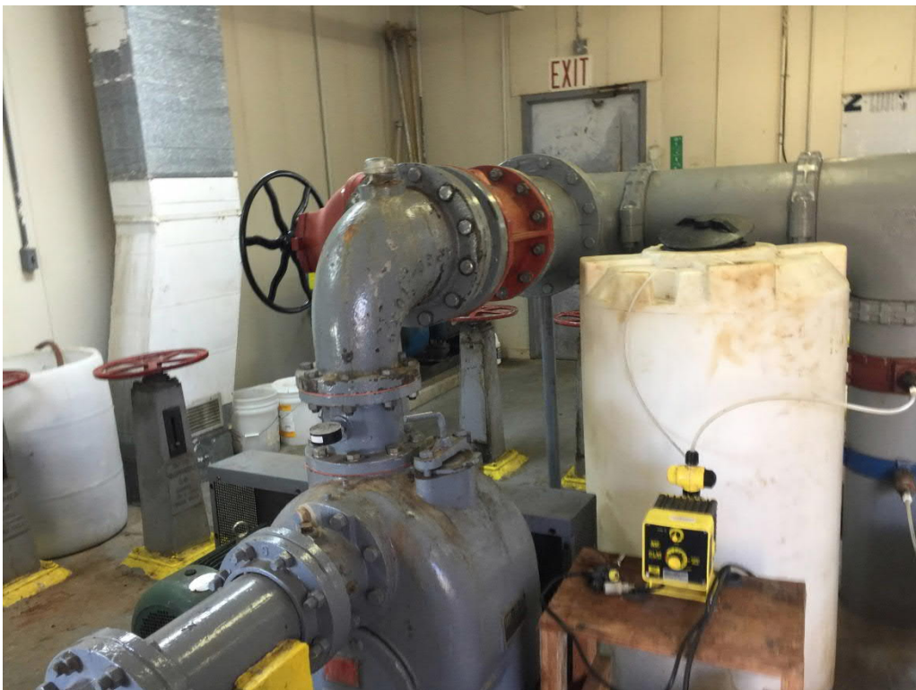
Figure 32: Phosphate Treatment Train - Intermediate Pump Station Piping
