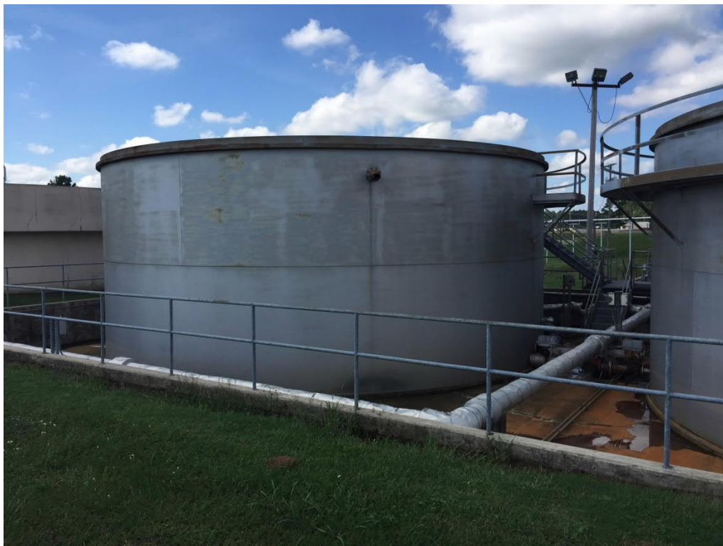
Figure 21: Chrome Treatment Train - Treated Water Storage Tanks
