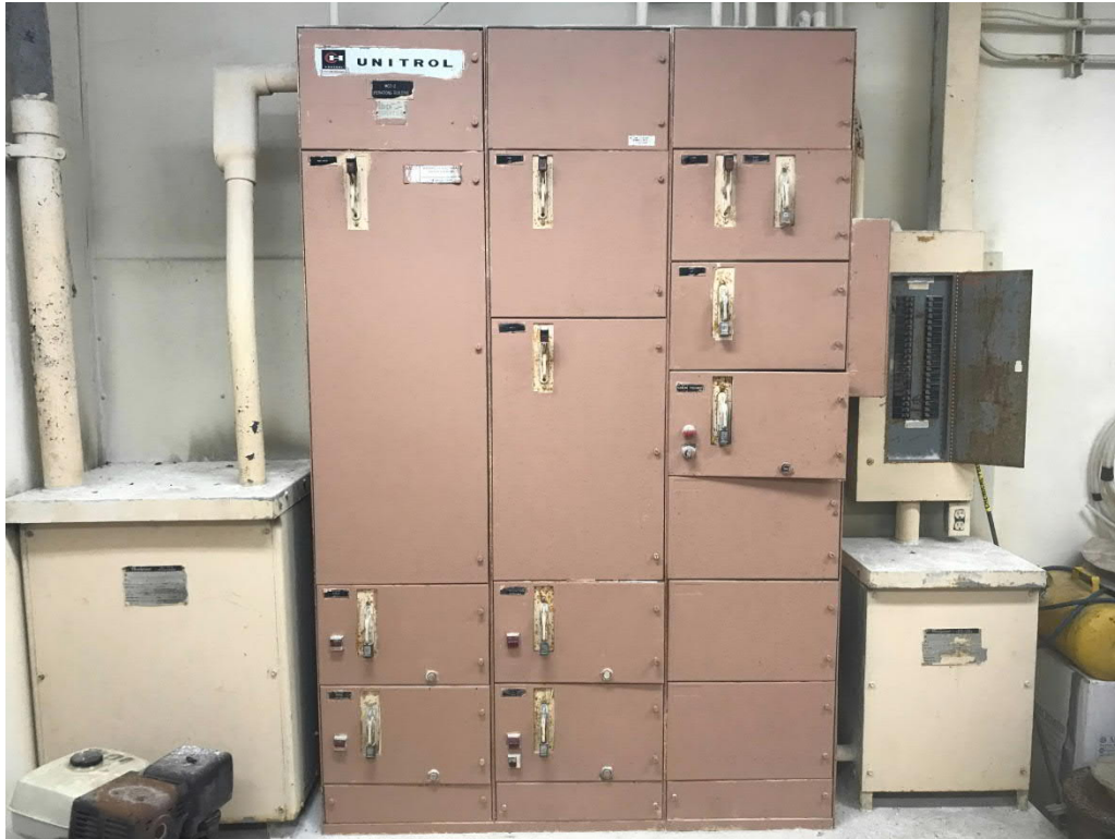
Figure1: Chrome Building 480V Motor Control Center
