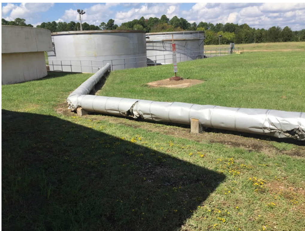
Figure 20: Chrome Treatment Train - Treated Water Storage Tanks
