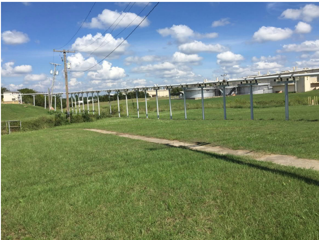
Figure 38: Phosphate Treatment Train - Grit Wash Pipe Line to Dewatering Beds
