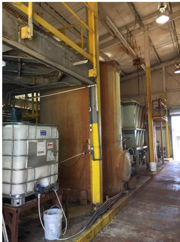
Figure 5: Chrome Treatment Train - UniPure Treatment System
