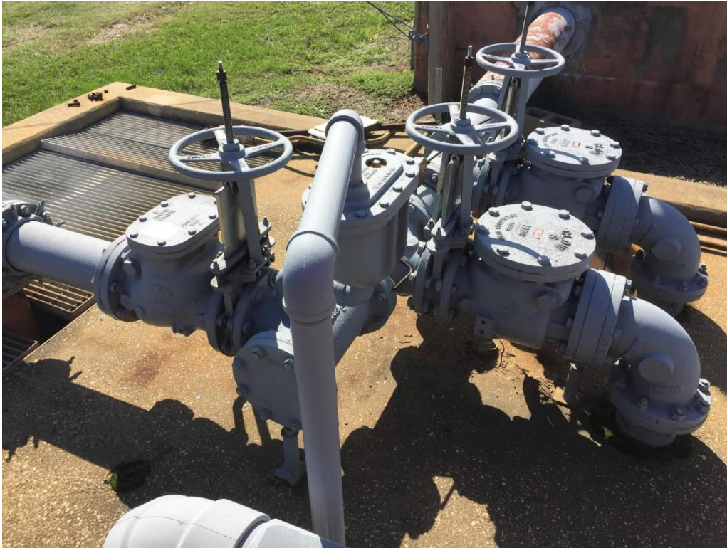
Figure1: Chrome Treatment Train - Lift Station
