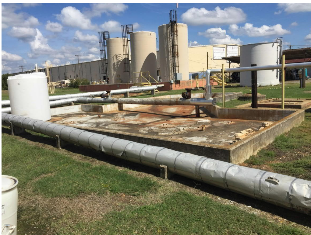
Figure 4: Chrome Treatment Train - Site Piping
