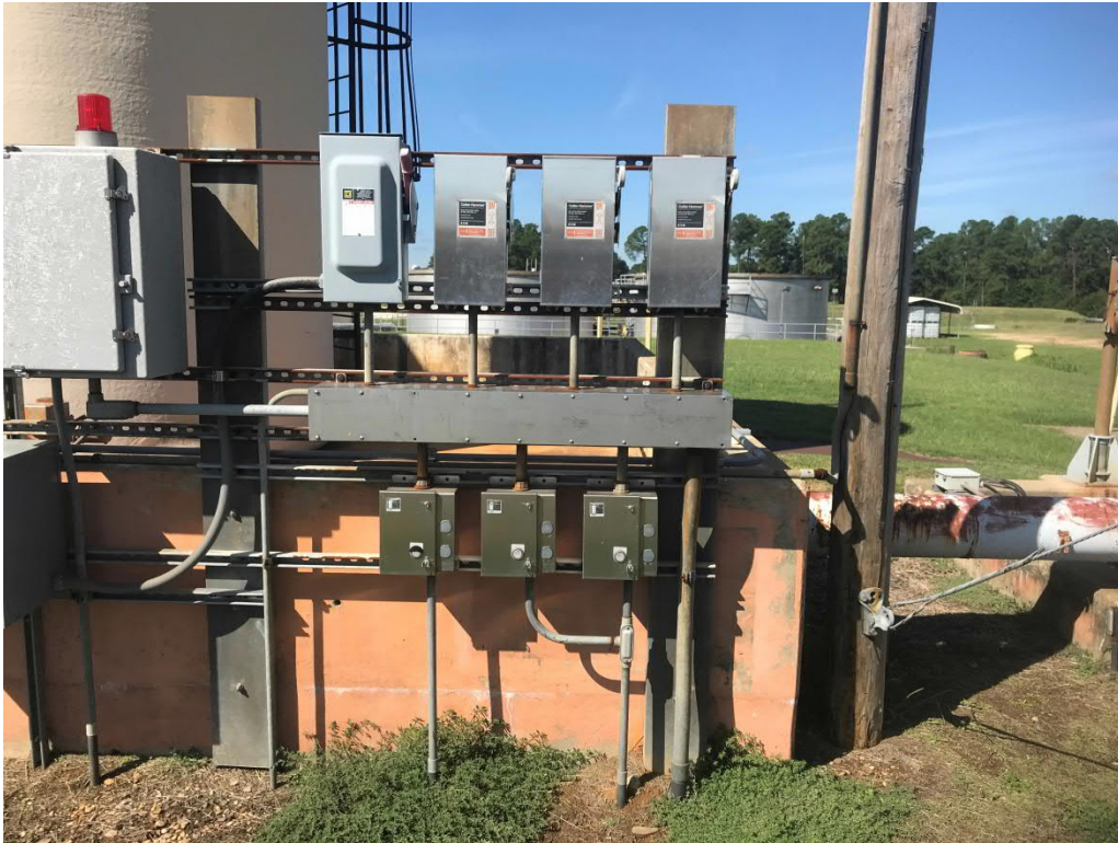
Figure 5: Chrome Lift Station electrical equipment
