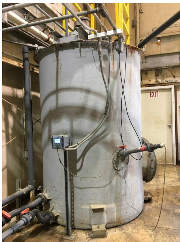
Figure 10: Chrome Treatment Train - pH Adjustment Tank
