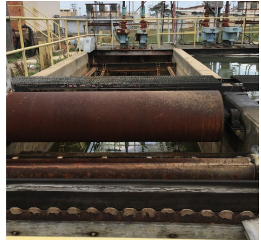
Figure 1: Oil Water Separator, out of service basin
