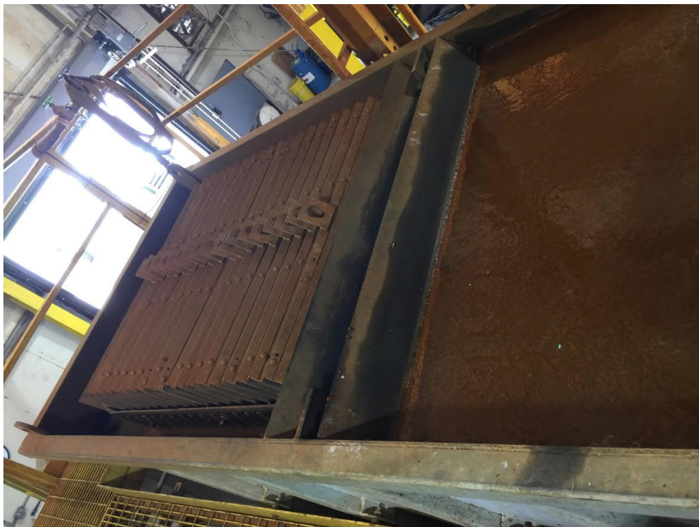
Figure 9: Chrome Treatment Train – Top of Inclined-Plate Clarifier
