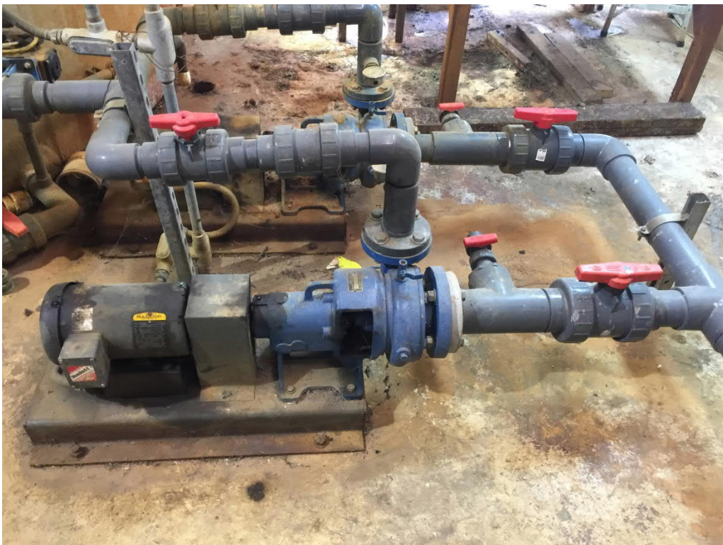
Figure 16: Chrome Treatment Train Tank Feed Pumps
