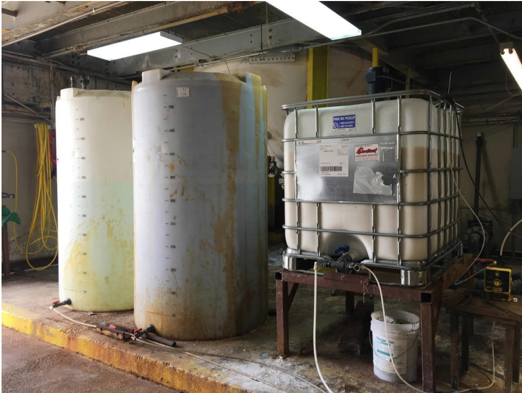
Figure 17: Chrome Treatment Train - Chemical Storage Tanks
