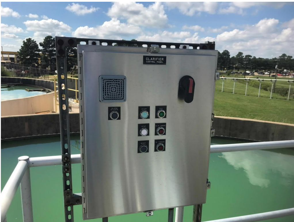
Figure 16: Rehabilitated Clarifier control panel
