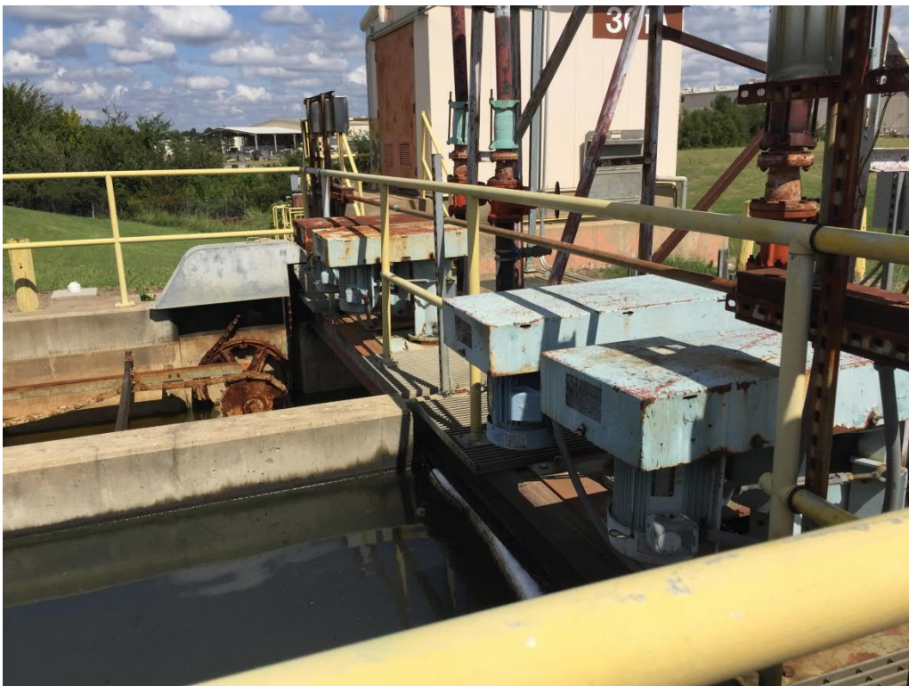
Figure 36: Phosphate Treatment Train - Oil-Water Separator Grit Pumps
