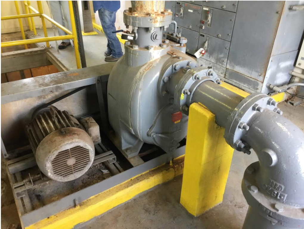
Figure 31: Phosphate Treatment Train - Intermediate Pump Station Pump
