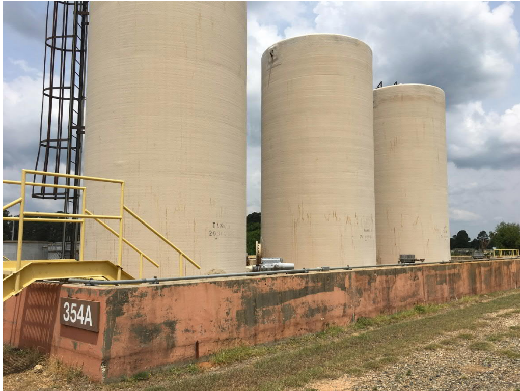
Figure 3: Chrome Treatment Train - Equalization Tanks
