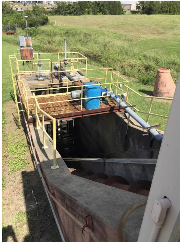
Figure 27: Phosphate Treatment Train - Influent Lift Station
