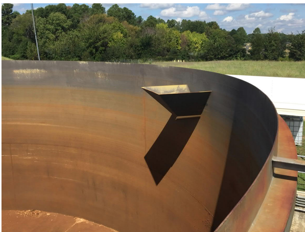
Figure 24: Chrome Treatment Train - Treated Water Storage Tank Overflow
