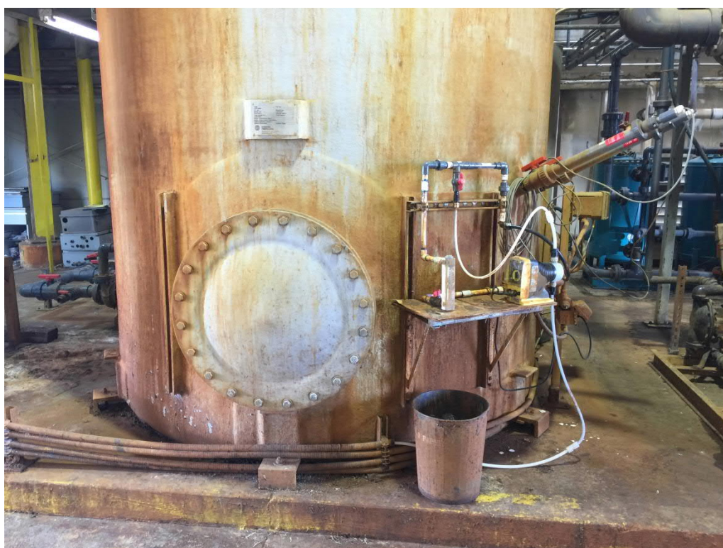
Figure 6: Chrome Treatment Train - Reactor Tank
