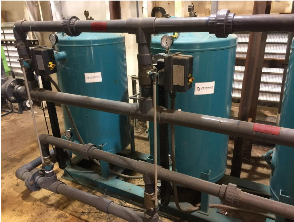
Figure 13: Chrome Treatment Train - Filters
