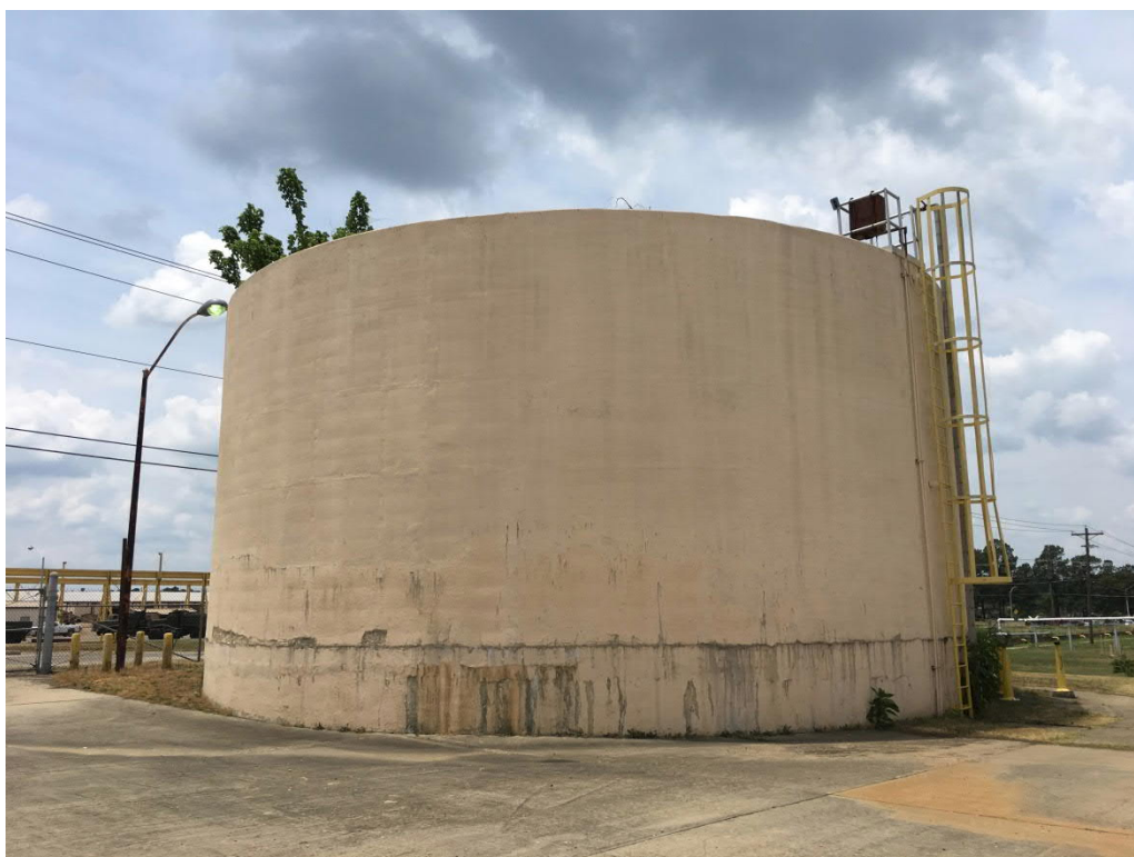
Figure 52: Phosphate Treatment Train - Unused Sludge Storage Tank
