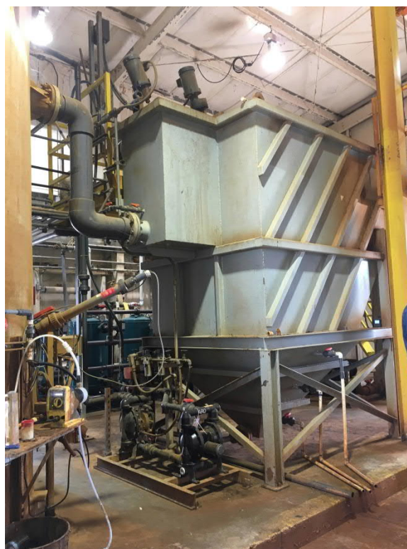
Figure 8: Chrome Treatment Train - Inclined-Plate Clarifier
