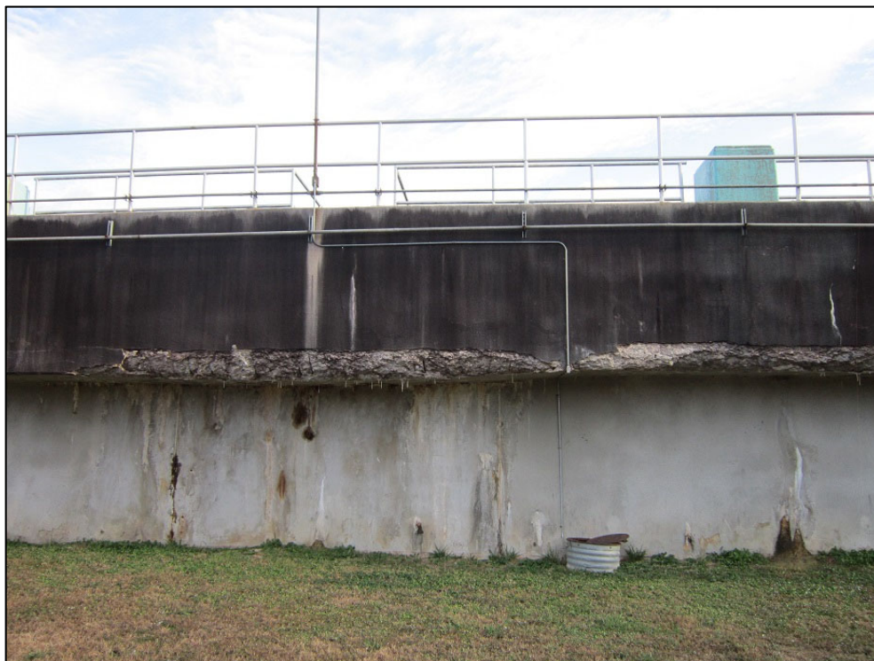
Figure 5-67: Observed Extreme Deflection on Basin Wall at Millwood WTP
