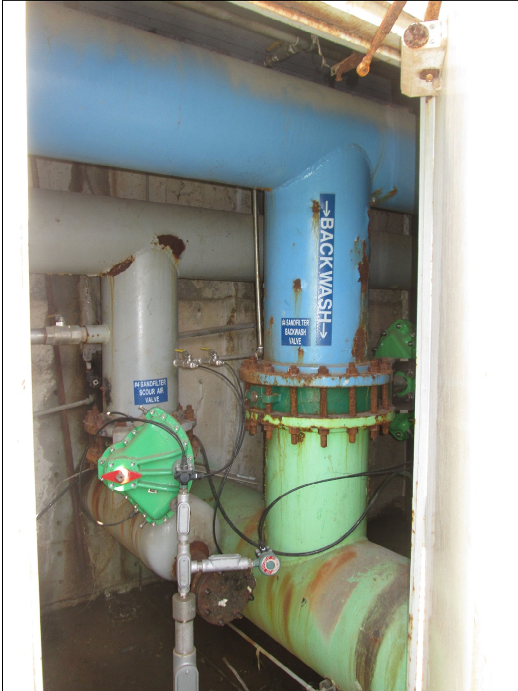
Figure 5-93: GPI WTP Filter Piping Showing Corrosion
