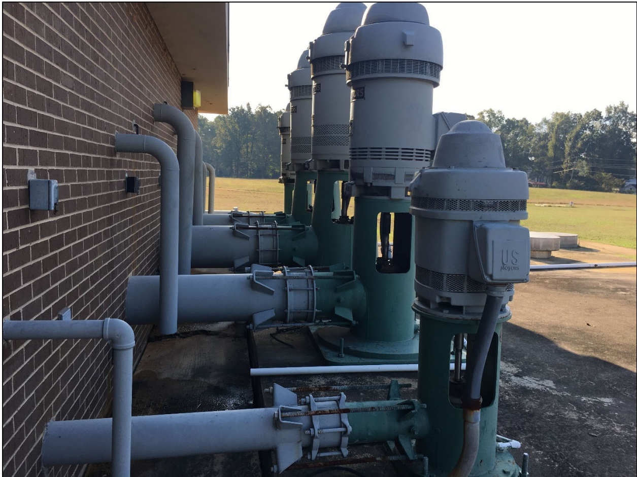
Figure 5-57: Millwood WTP High Service Pump Station
