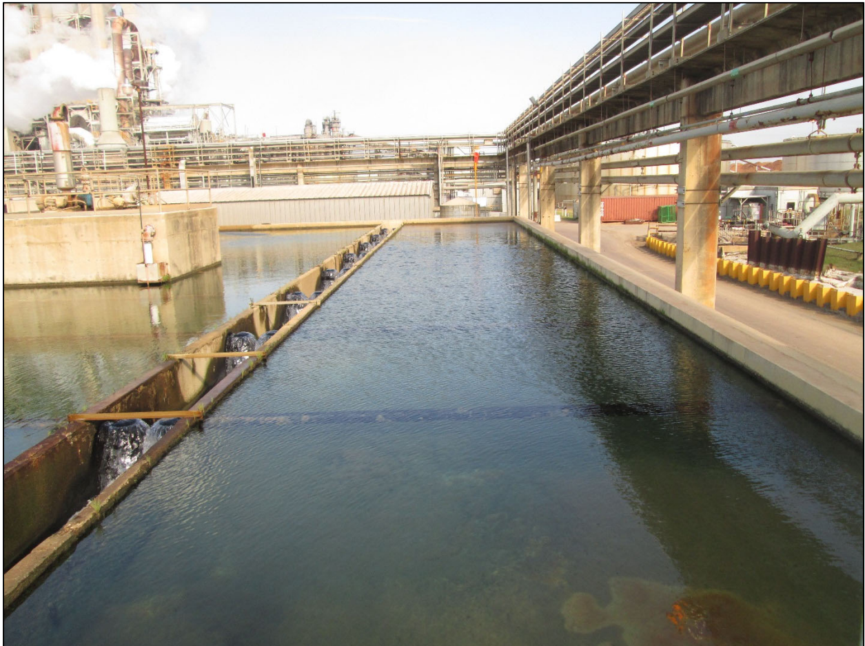
Figure 5-89: GPI WTP High Rate Clarifiers Shown Working Well.
