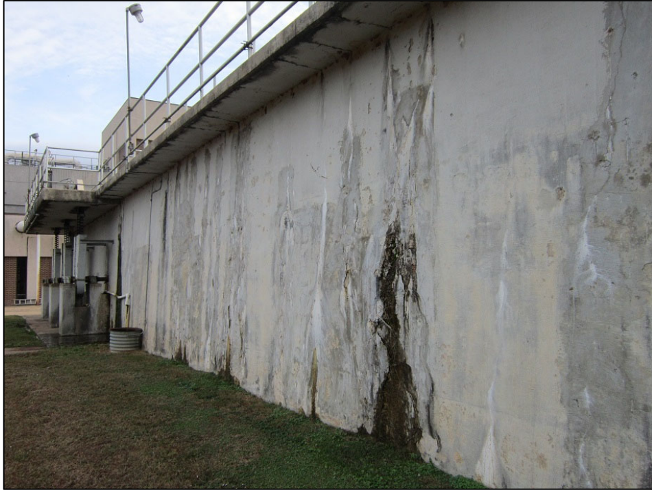
Figure 5-61: Observed Cracking on Basin Wall at Millwood WTP
