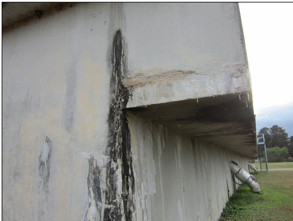
Figure 5-60: Observed Cracking on Basin at Millwood WTP
