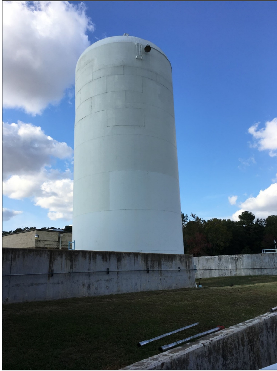
Figure 5-20: New Boston Road WTP Backwash Tank where Outside Condition of Tank Appears Good
