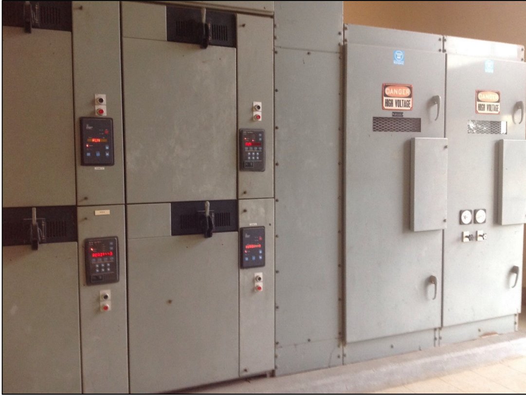
Figure 5-72: High Service Switchgear at Millwood WTP
