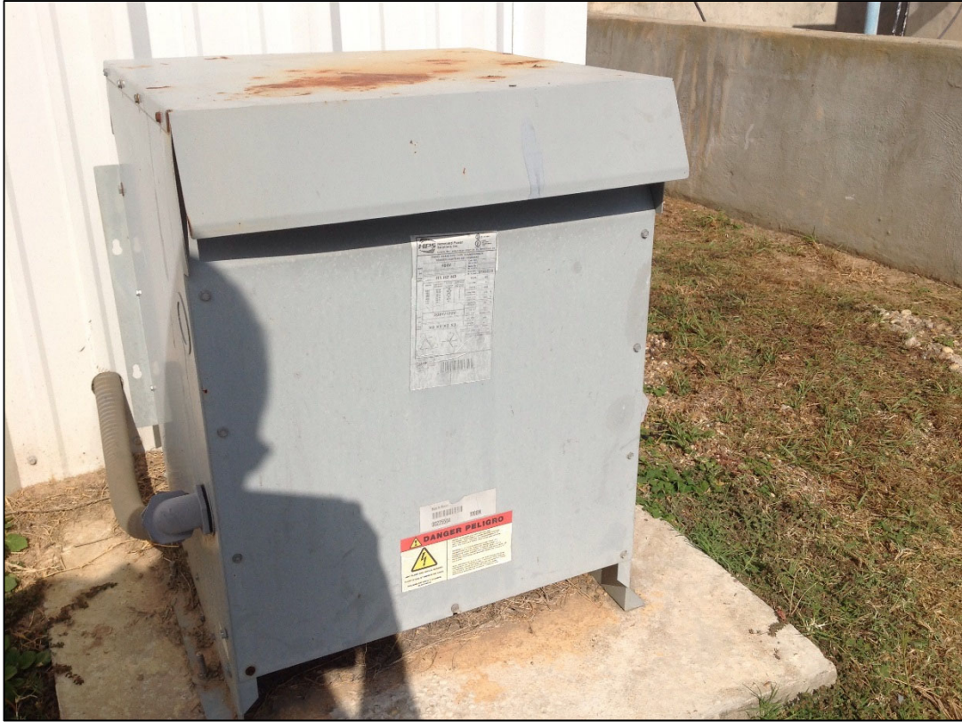
Figure 5-35: Example of a 480V Transformer (at Caustic Building) at New Boston Road WTP
