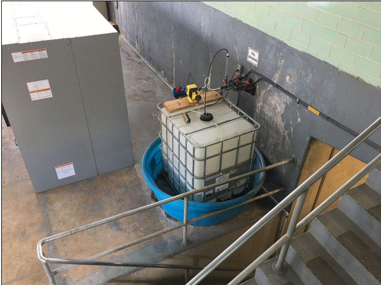
Figure 5-28: New Boston Road WTP Polyphosphate Feed System
