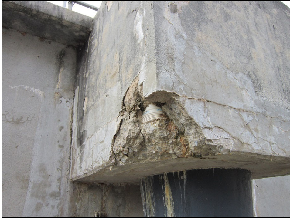
Figure 5-66: Observed Extreme Concrete Spalling and Erosion (note lack of rebar) on Structure at Millwood WTP
