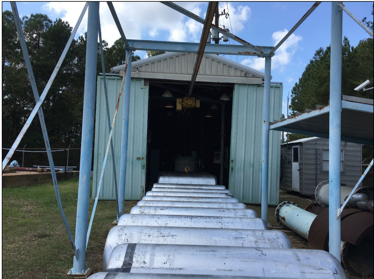
Figure 5-77: GPI WTP Intake Pipeline Chlorination Handling System
