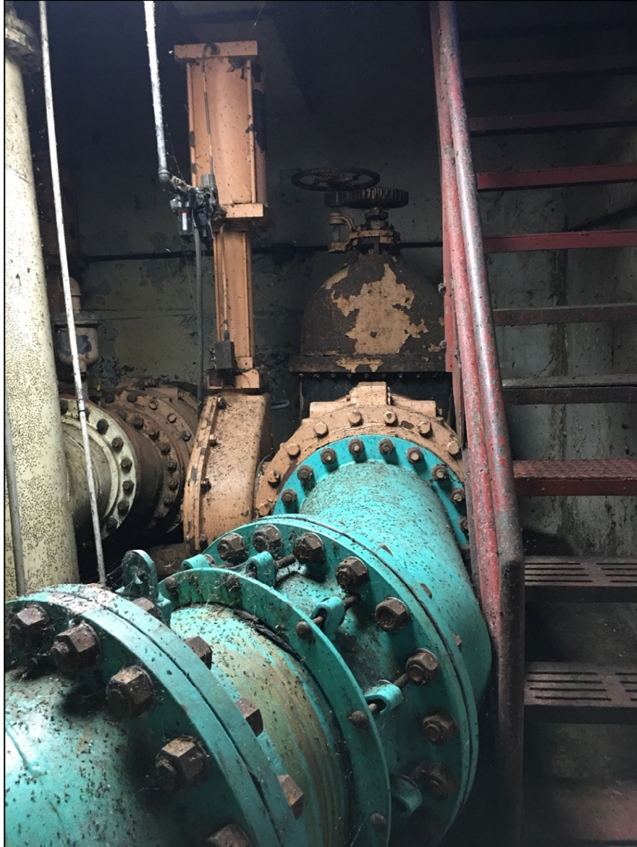
Figure 5-12: Discharge Piping in Raw Water Pump Station showing coating in need of repair and other wear and tear
