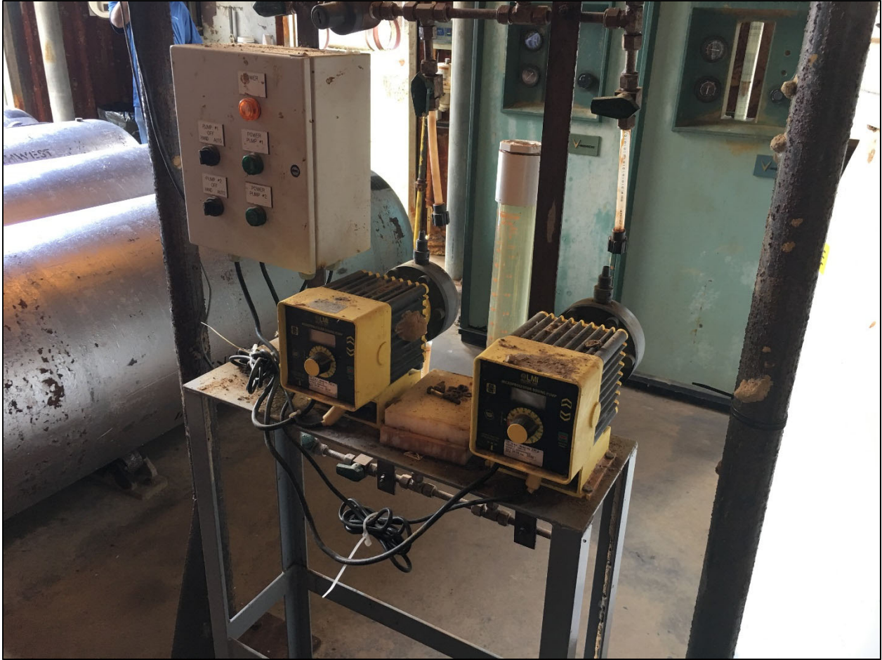
Figure 5-80: GPI WTP Intake Pipeline Sodium Permanganate Feed System
