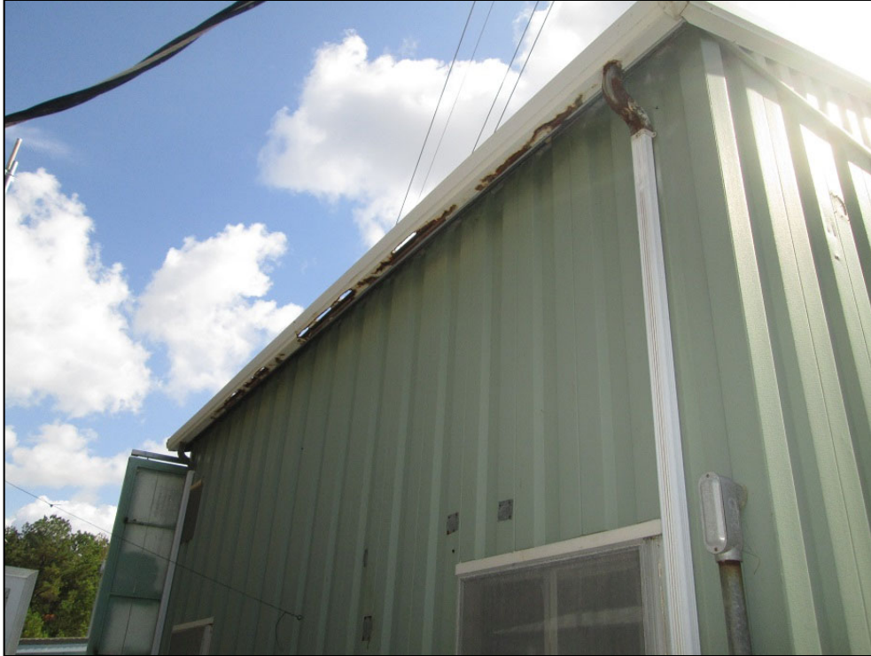
Figure 5-84: Prefabricated Chlorine Building at GPI Showing Corrosion in Gutters
