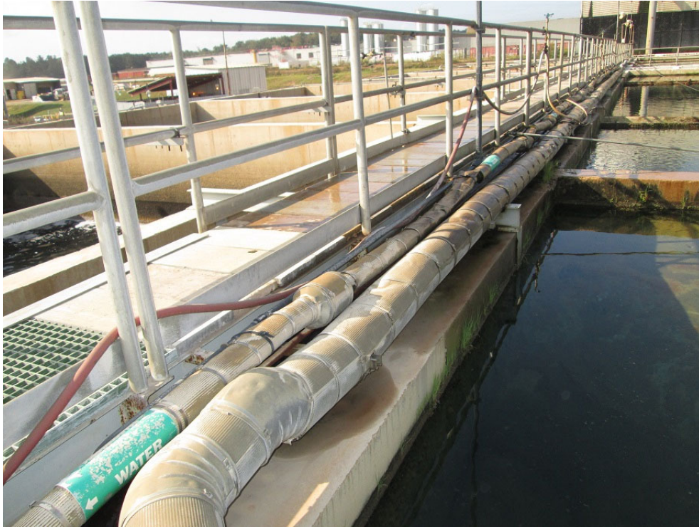
Figure 5-109: Example of Pipe Deflection at GPI WTP
