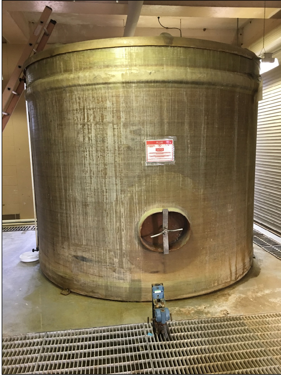
Figure 5-49: Millwood WTP Primary Coagulant Tank
