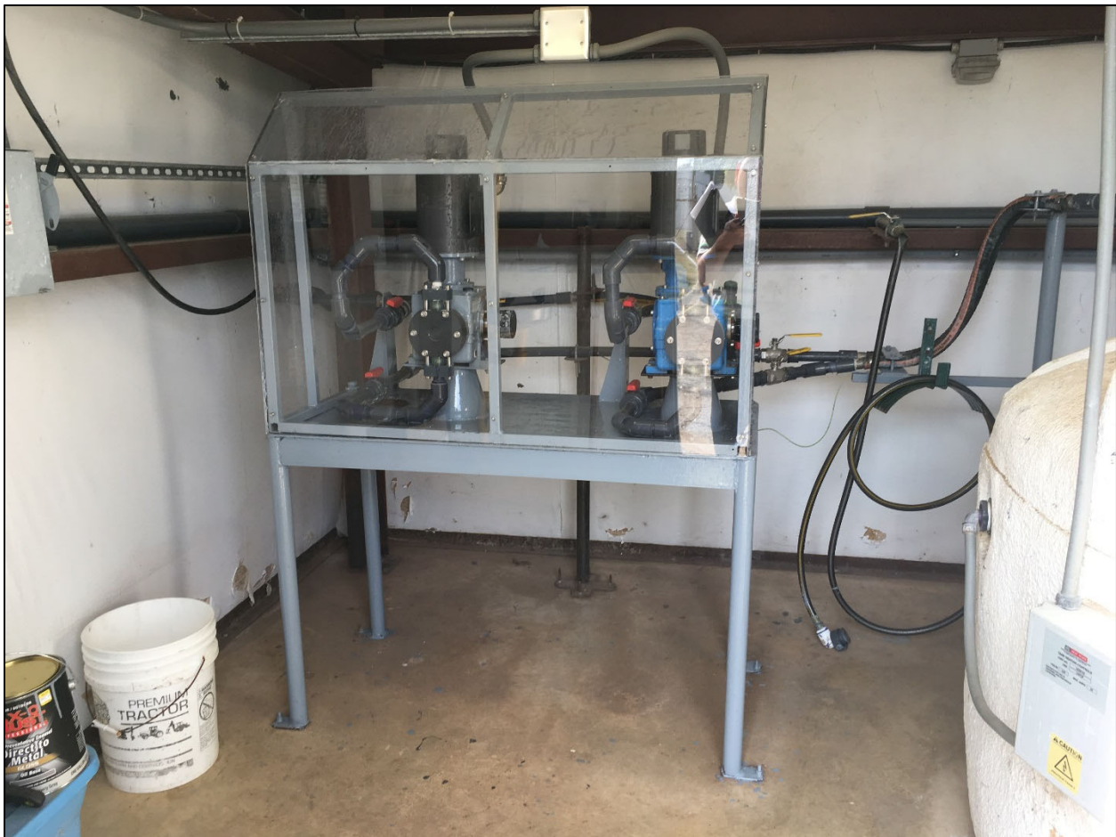
Figure 5-24: New Boston Road WTP Sodium Hydroxide Feed System
