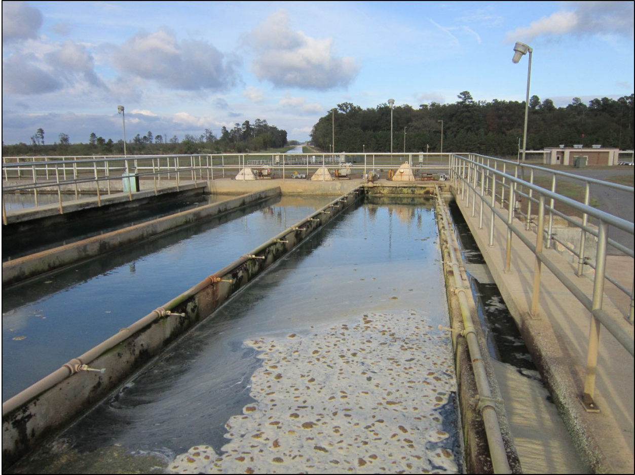
Figure 5-41: Millwood WTP Flocculation Basins
