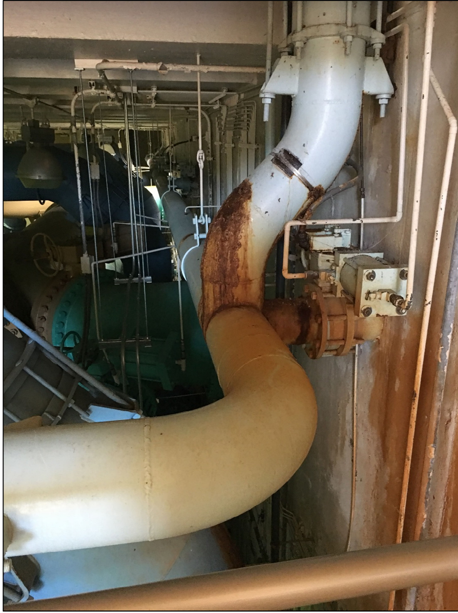
Figure 5-46: Millwood WTP Filter Gallery Piping Showing Corrosion
