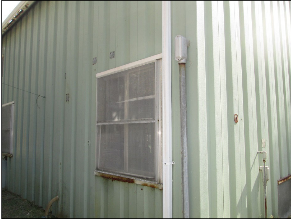
Figure 5-85: Prefabricated Chlorine Building at GPI Showing Corrosion on Window
