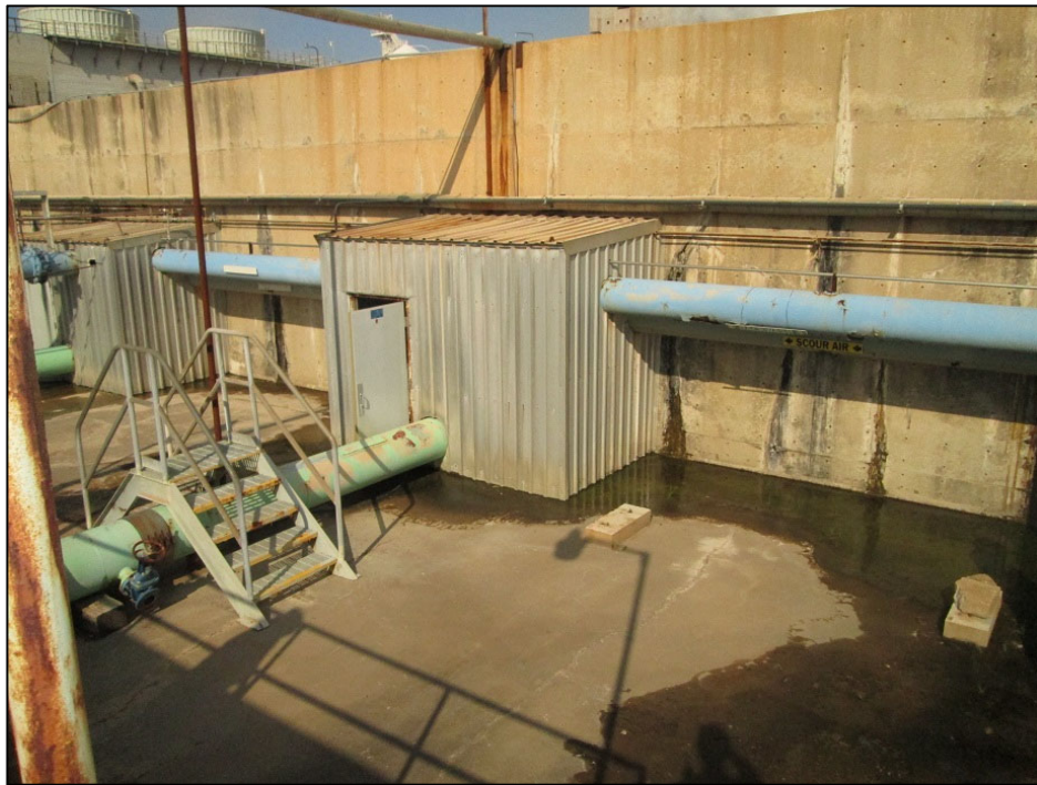
Figure 5-106: Cracks in Basin Wall and Resulting Leakage and Corrosion at GPI WTP
