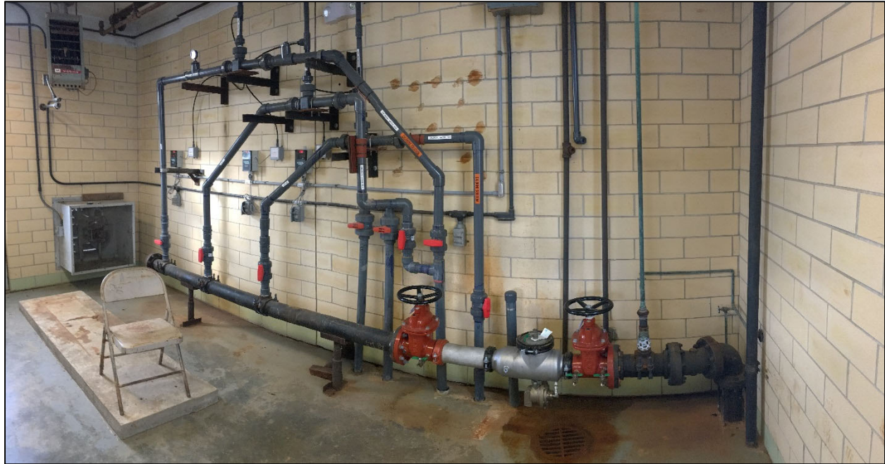
Figure 5-25: New Boston Road WTP Chlorine Dioxide Feed System
