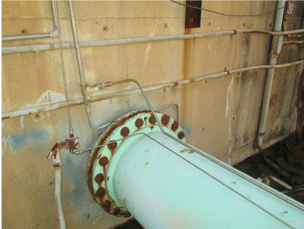
Figure 5-111: Example of Corrosion at Pipe Connections at GPI WTP
