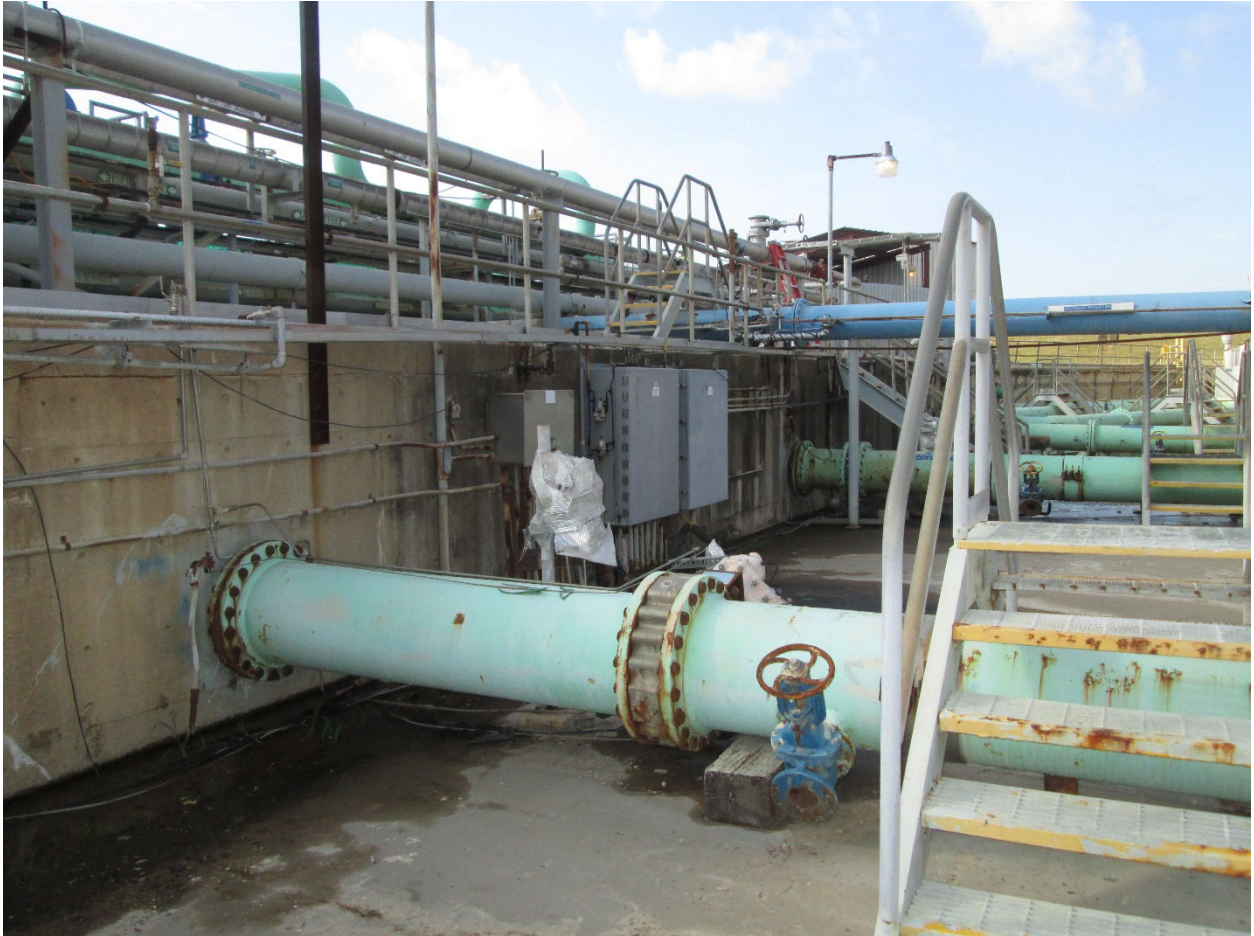
Figure 5-91: GPI WTP Filter Effluent Piping Showing Corrosion
