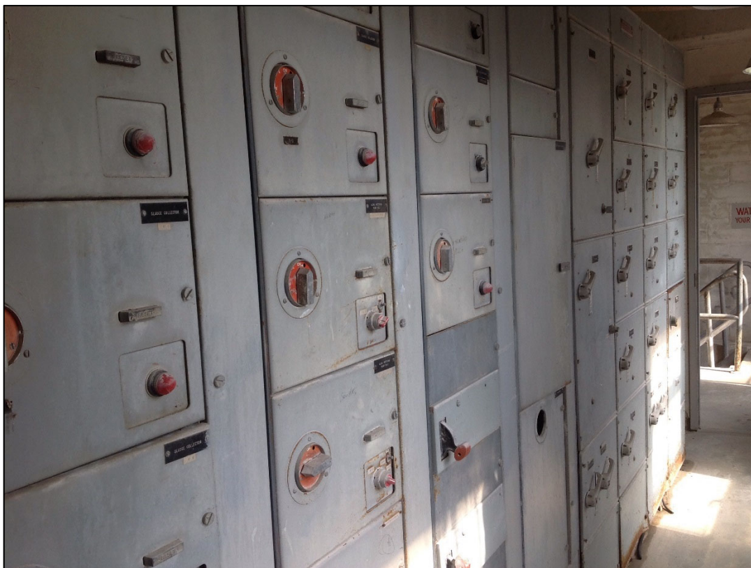
Figure 5-34: Main MCC at New Boston Road WTP
