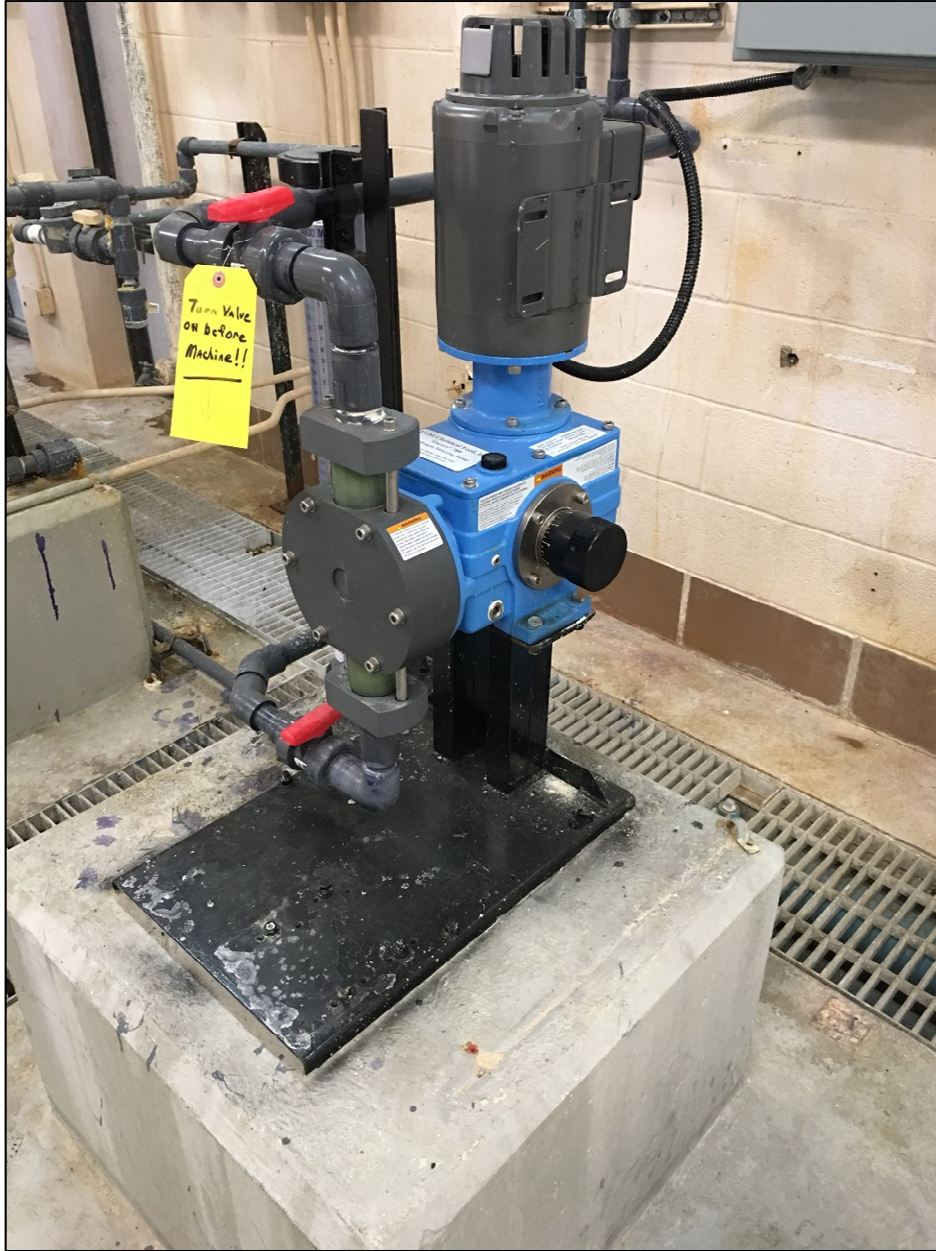
Figure 5-50: Millwood WTP Primary Coagulant Feed Pumps
