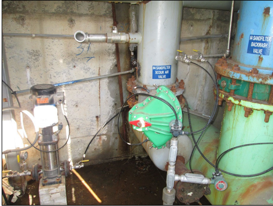
Figure 5-107: Crack in Basin Wall and Resulting Leakage and Corrosion at GPI WTP
