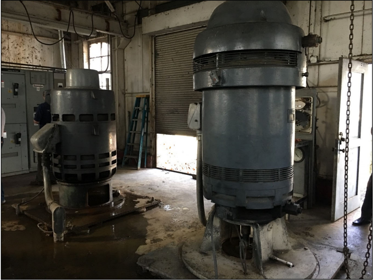
Figure 5-10: Vertical Turbine Pump Motors inside the Raw Water Pump Station showing exposure to moisture and other elements
