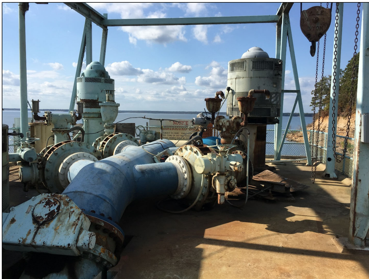
Figure 5–75: GPI WTP Intake Pump Station Pumps and Piping Showing Deficient Coatings
