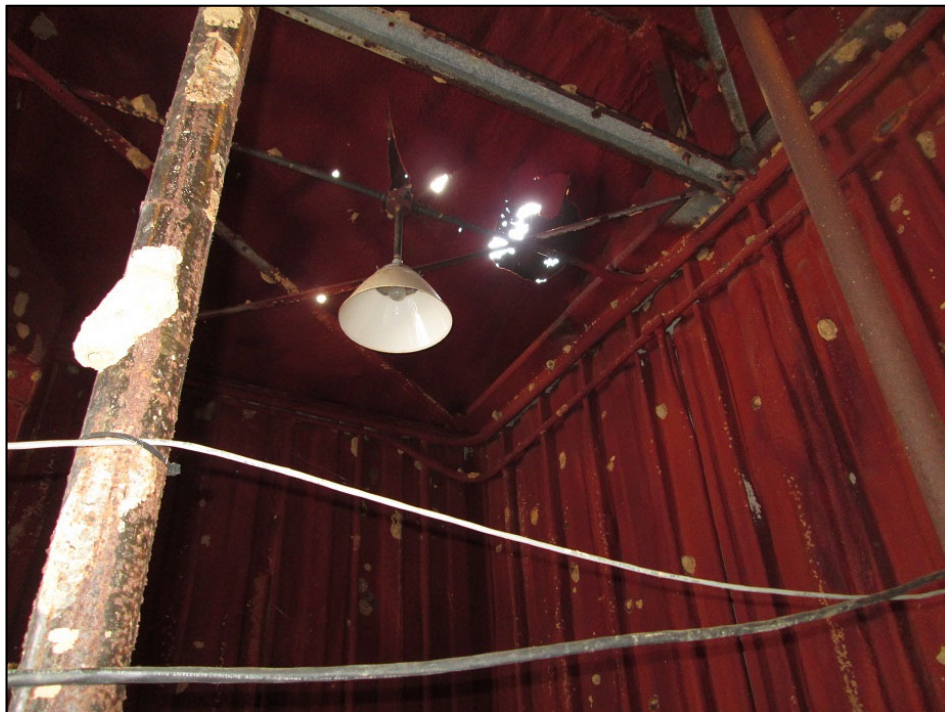
Figure 5-83: Prefabricated Chlorine Building at GPI Showing Corrosion and Opening in Roof
