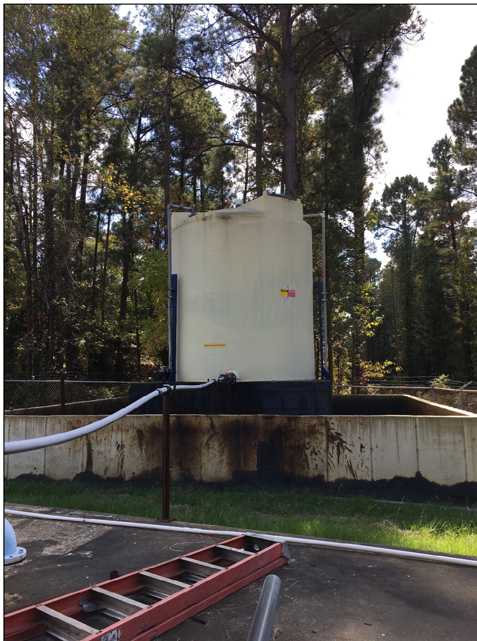
Figure 5-79: GPI WTP Intake Pipeline Sodium Permanganate Tank
