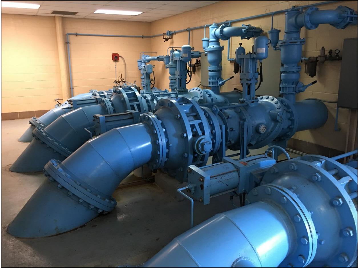
Figure 5-58: Millwood WTP High Service Pump Station Discharge Piping Shown in Good Condition
