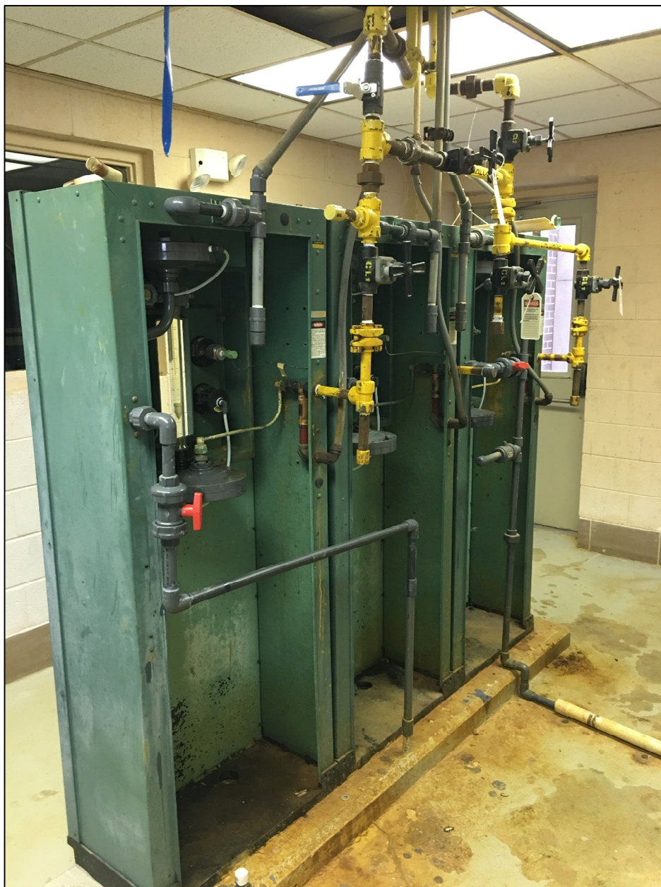
Figure 5-47: Millwood WTP Chlorinators
