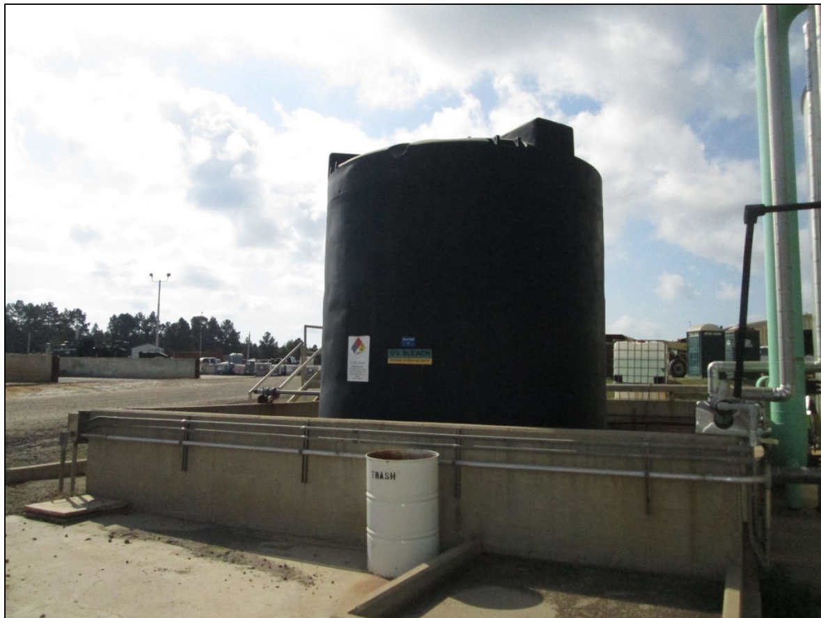
Figure 5-99: GPI WTP Sodium Hypochlorite Tank Shown in Good Condition
