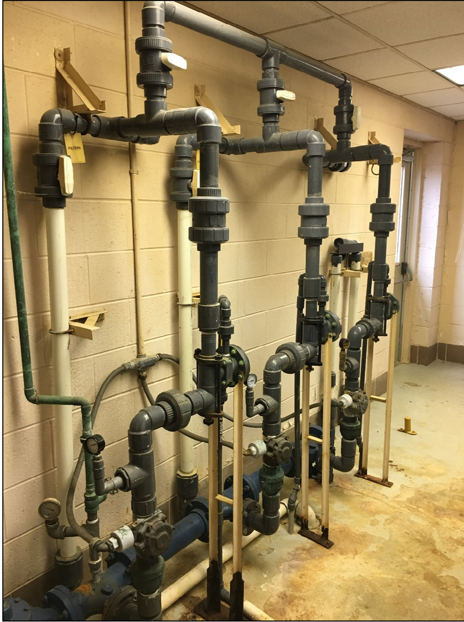
Figure 5-48: Millwood WTP Chlorine Feed System
