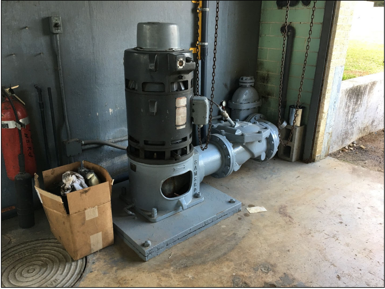
Figure 5-21: New Boston Road WTP Backwash Pump
