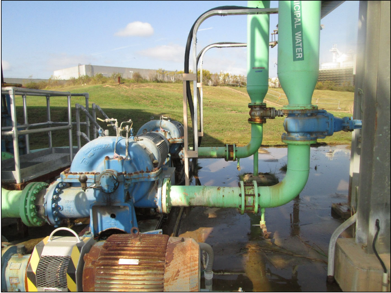
Figure 5-98: GPI WTP Potable Water Pumps and Piping Showing Corrosion
