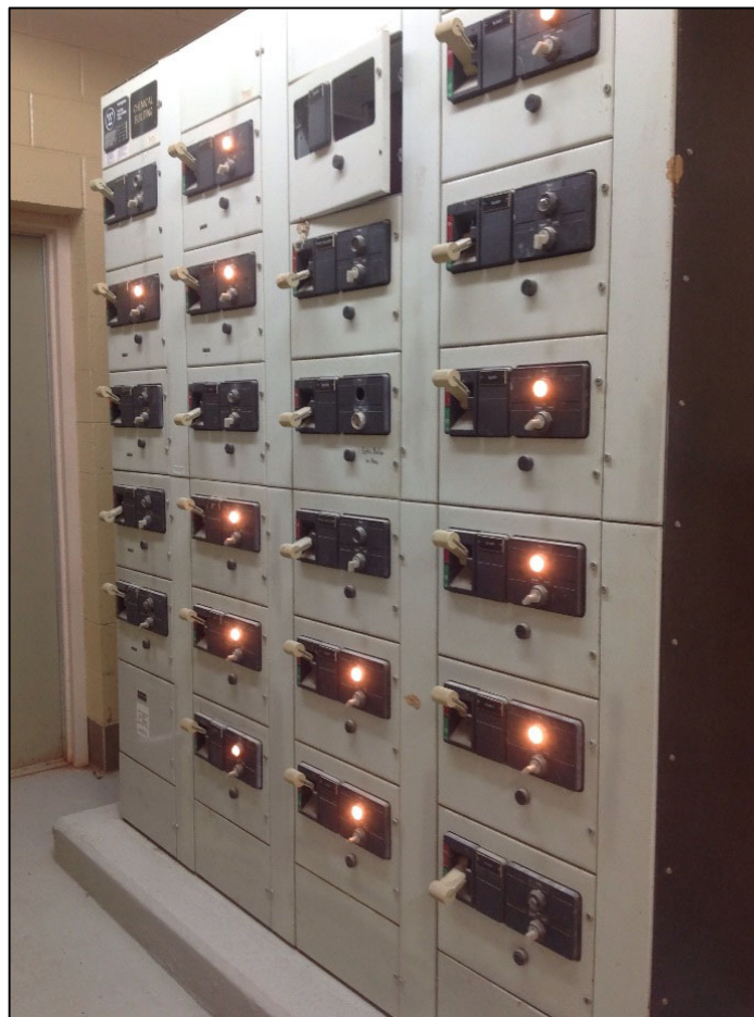
Figure 5-71: Chemical Building MCC at Millwood WTP in Fair Condition
