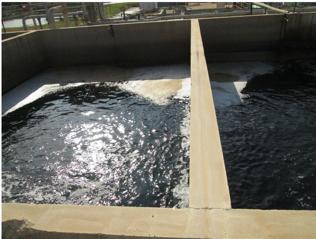
Figure 5-90: GPI WTP Sand Filters Shown Working Well.
