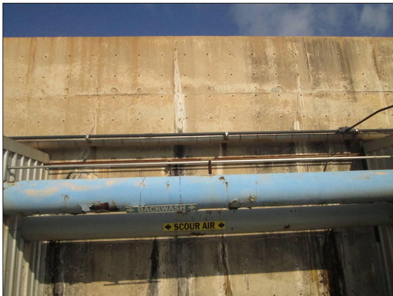
Figure 5-92: GPI WTP Filter Piping Showing Corrosion
