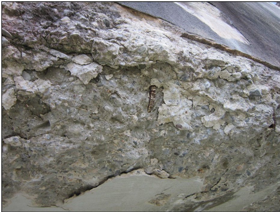
Figure 5-65: Observed Exposed Rebar and Concrete Spalling on Structure at Millwood WTP
