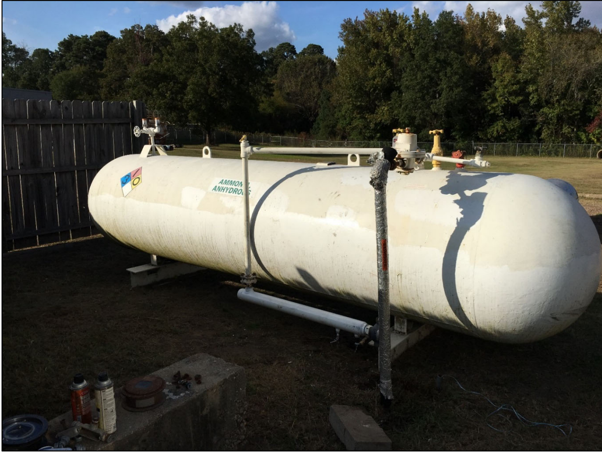
Figure 5-26: New Boston Road WTP Ammonia Tank
