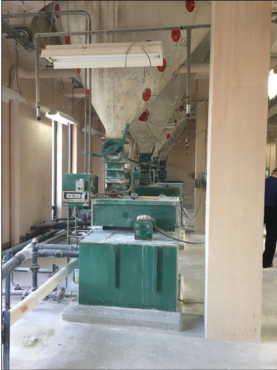
Figure 5-51: Millwood WTP Lime Slakers
