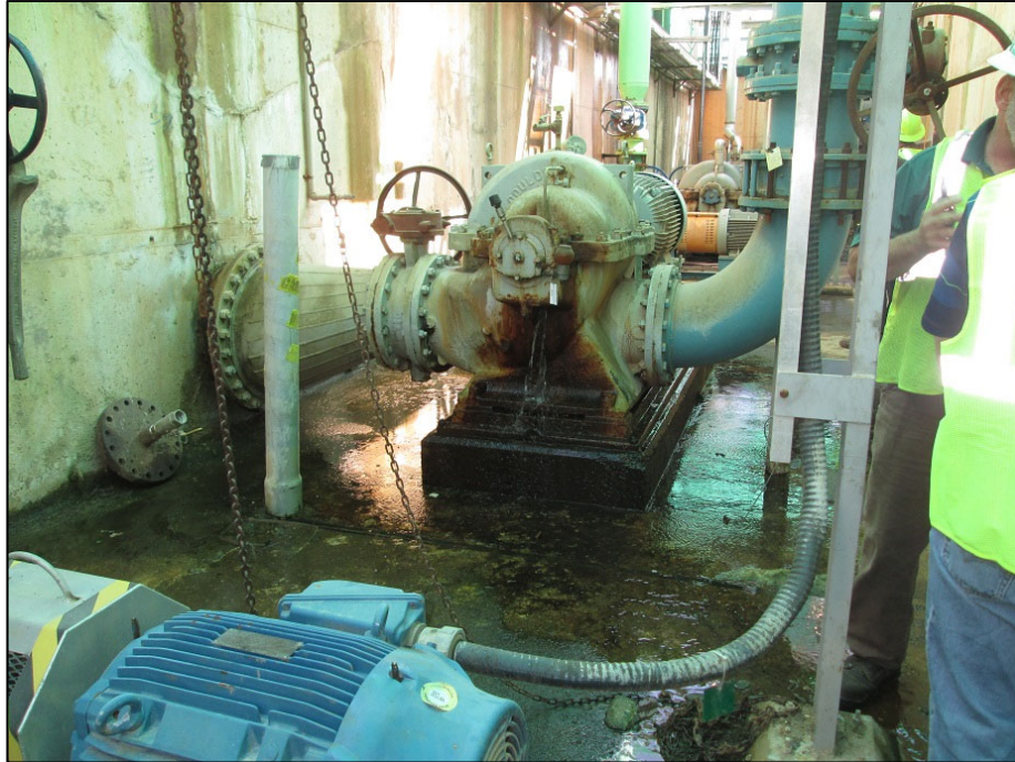
Figure 5-101: Pump at GPI WTP Showing Leakage
