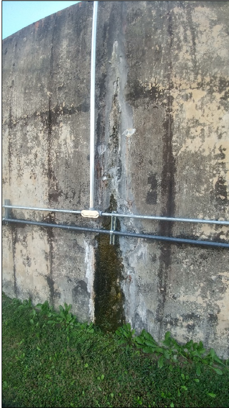
Figure 5-30: Observed Effects of Water Leakage along Basin Wall at New Boston Road WTP
