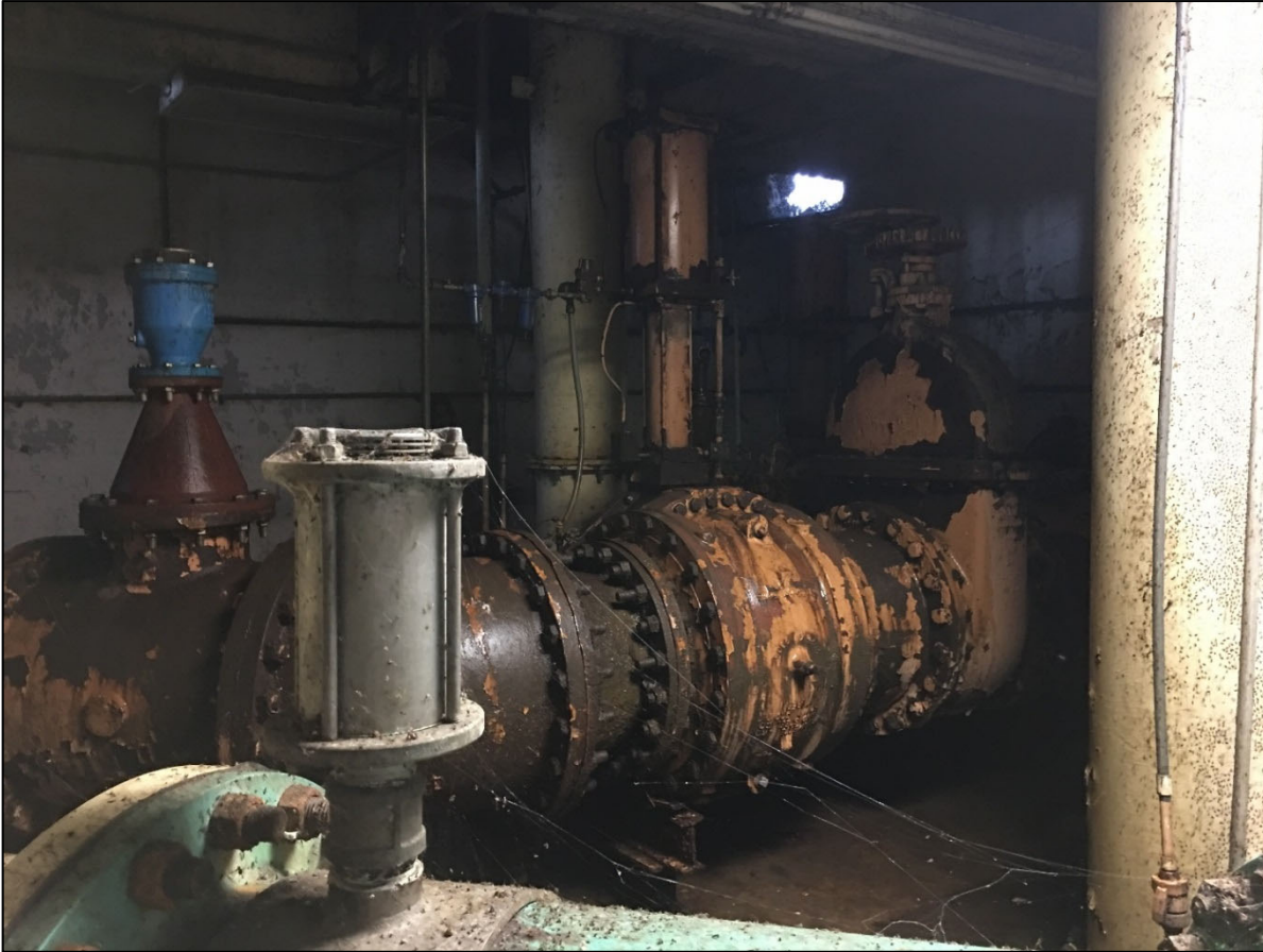
Figure 5-11: Discharge Piping in Raw Water Pump Station showing moist environment and lack of coating.
