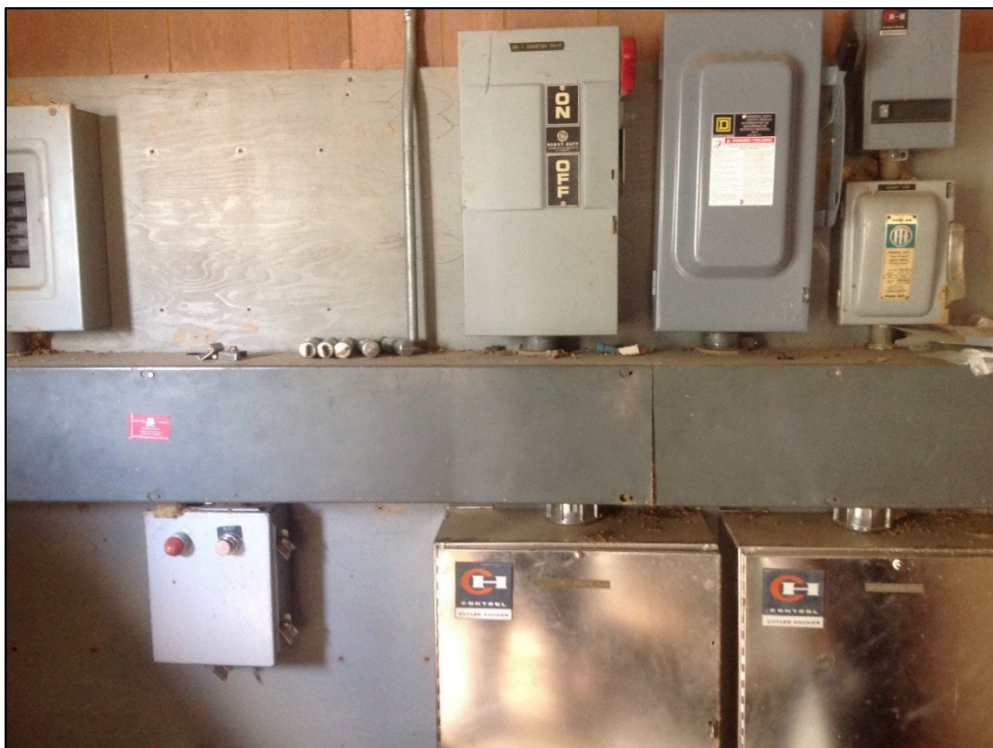
Figure 5-87: VFDs at GPI Intake Recently Replaced
