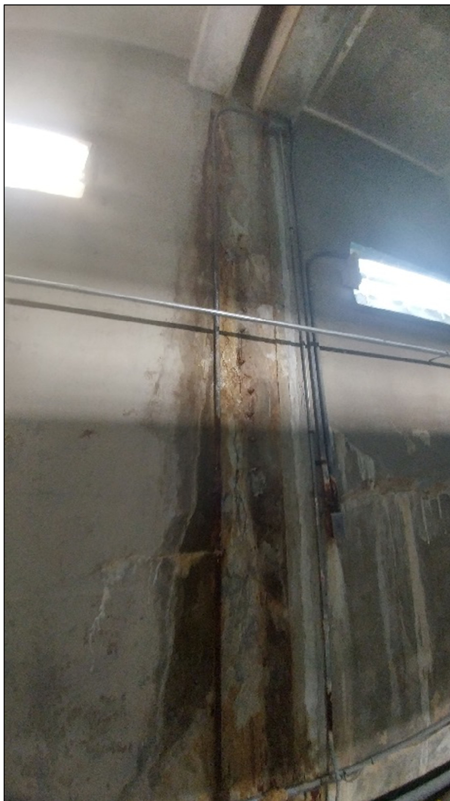
Figure 5-31: Observed Effects of Water Leakage within New Boston Road WTP
