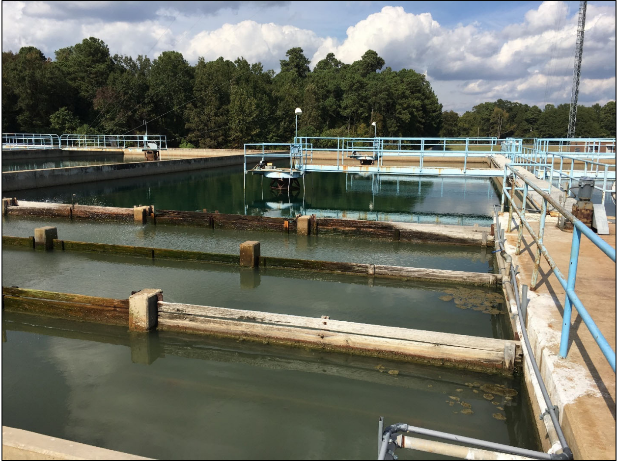
Figure 5-16: New Boston Road WTP Flocculation/Sedimentation Basins showing baffles and sludge collectors that are past their expected useful life
