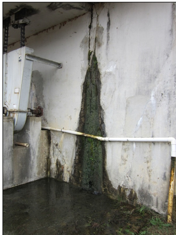
Figure 5-62: Observed Cracking and Leakage on Basin Wall at Millwood WTP
