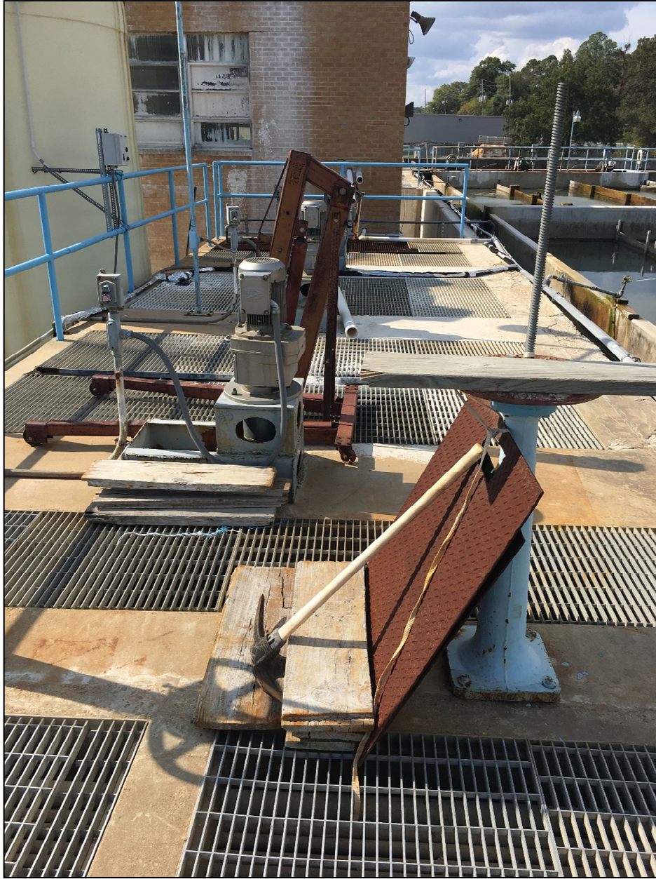
Figure 5-15: New Boston Road WTP Flash Mix Basin showing mixers that are aged past their useful life
