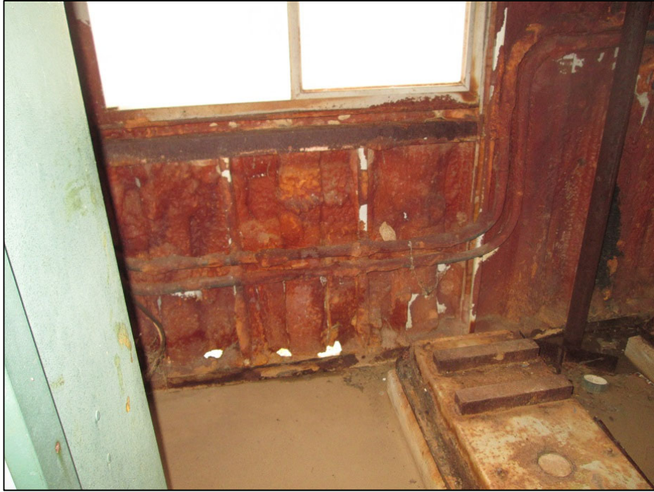
Figure 5-82: Prefabricated Chlorine Building at GPI Showing Rust and Corrosion
