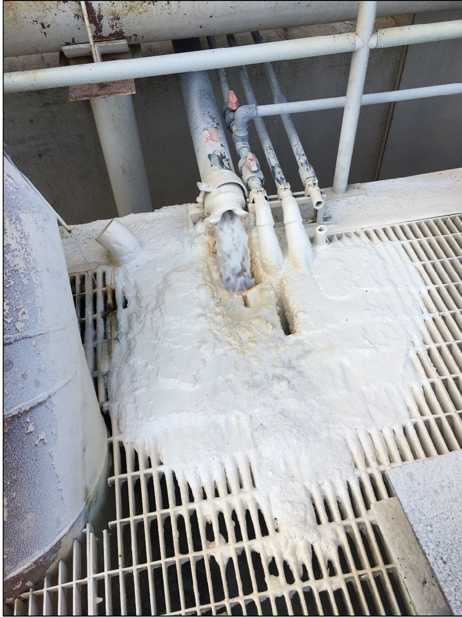
Figure 5-52: Millwood WTP Lime Injection
