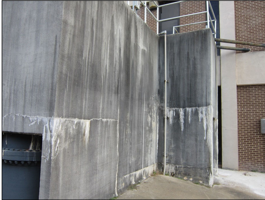
Figure 5-63: Observed Cracking in Basin Walls; No Apparent Expansion Joints at Millwood WTP
