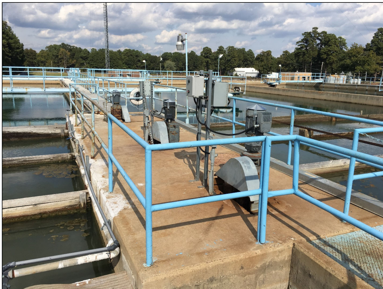
Figure 5-17: New Boston Road WTP Flocculators that are past their expected useful life
