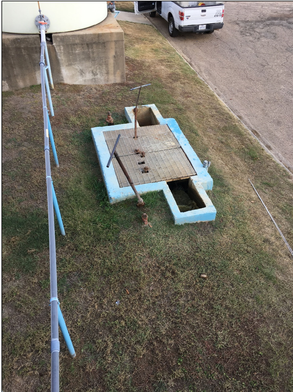
Figure 5-29: New Boston Road WTP Residuals Collection Vault
