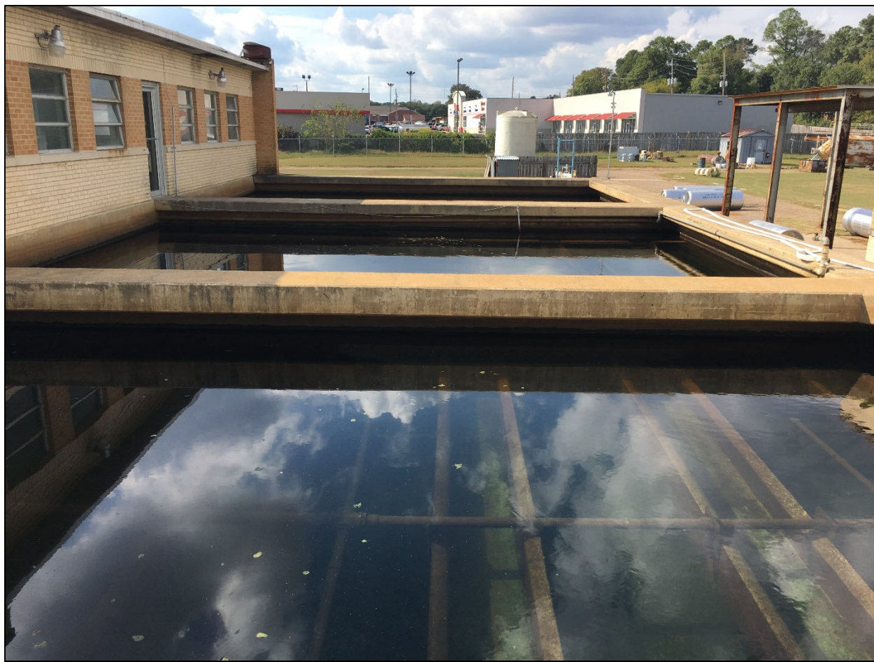
Figure 5-19: New Boston Road WTP Filters showing aged launders
