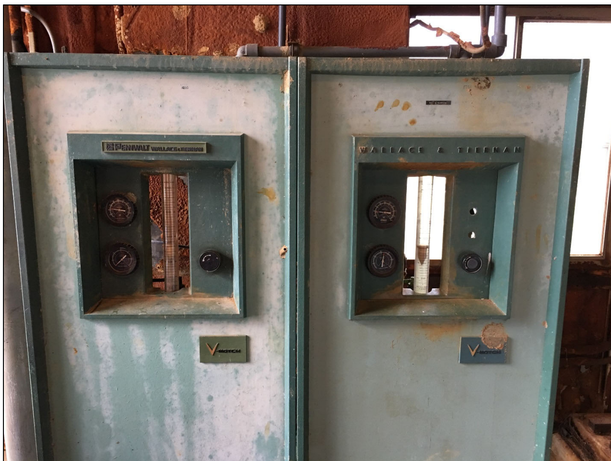
Figure 5-78: GPI WTP Intake Pipeline Chlorinators
