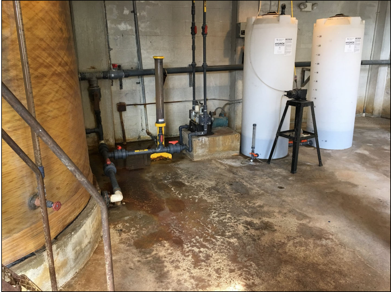
Figure 5-23: New Boston Road WTP Primary Coagulant Feed System
