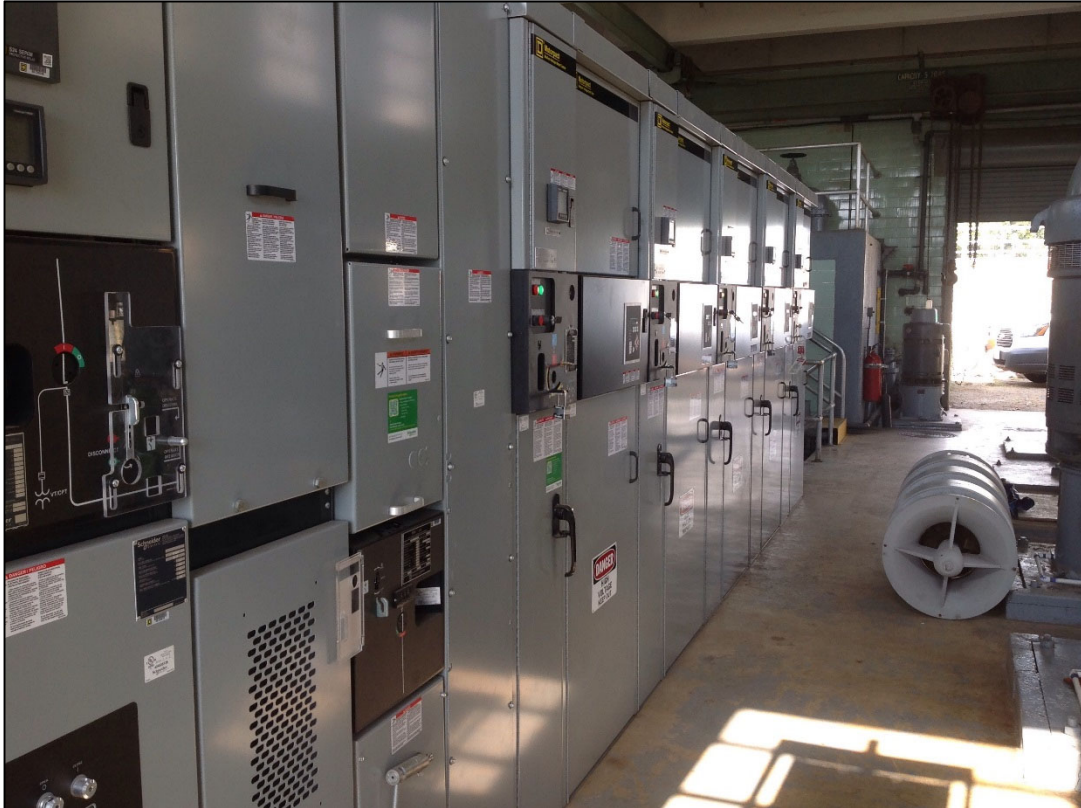
Figure 5-33: Main Switchgear at New Boston Road WTP
