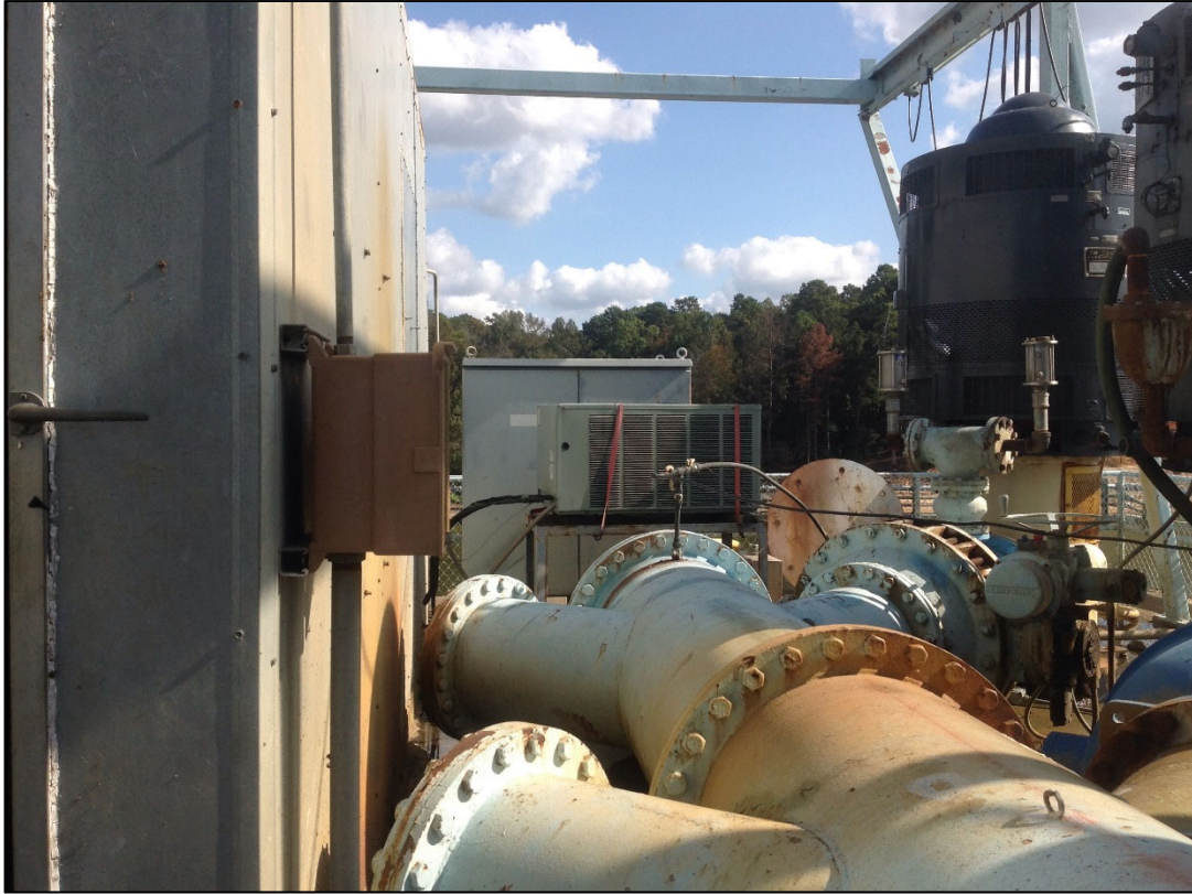
Figure 5-88: Outside Motors at GPI Intake Showing Corrosion and Some Out-of-Service Motors
