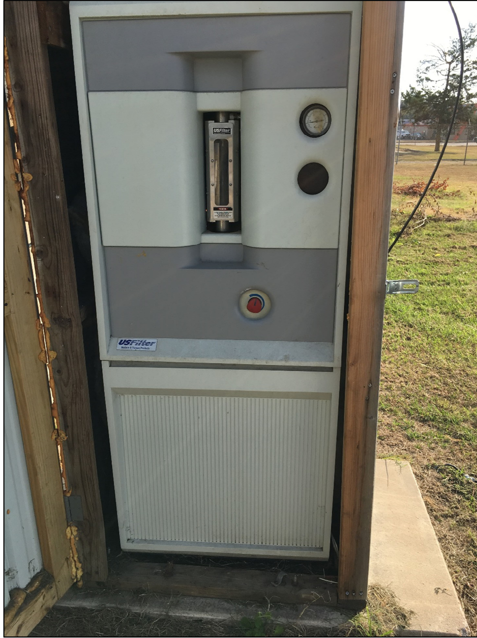
Figure 5-27: New Boston Road WTP Ammoniator
