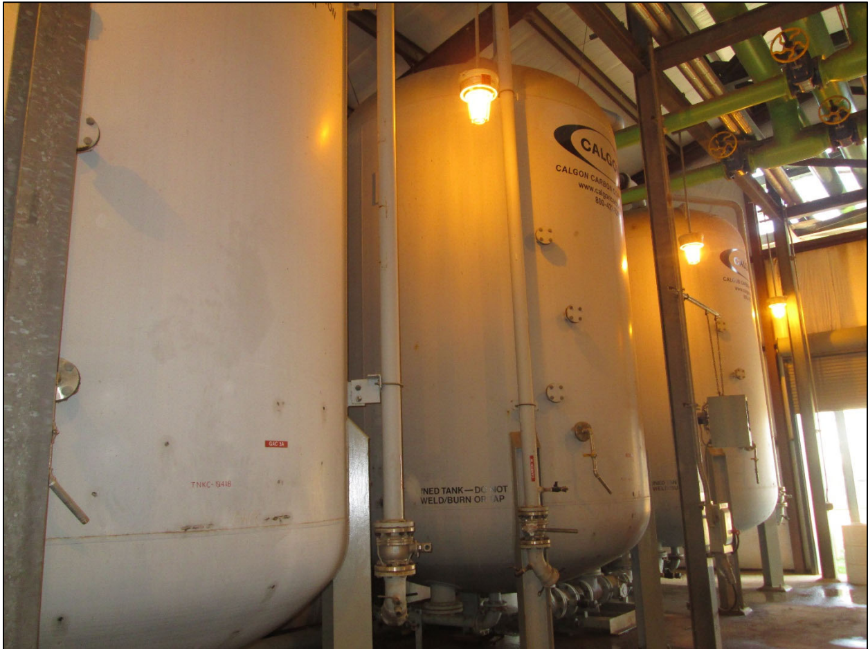
Figure 5-96: GPI WTP GAC Contactors Showing Potential Needs for Coating Repair
