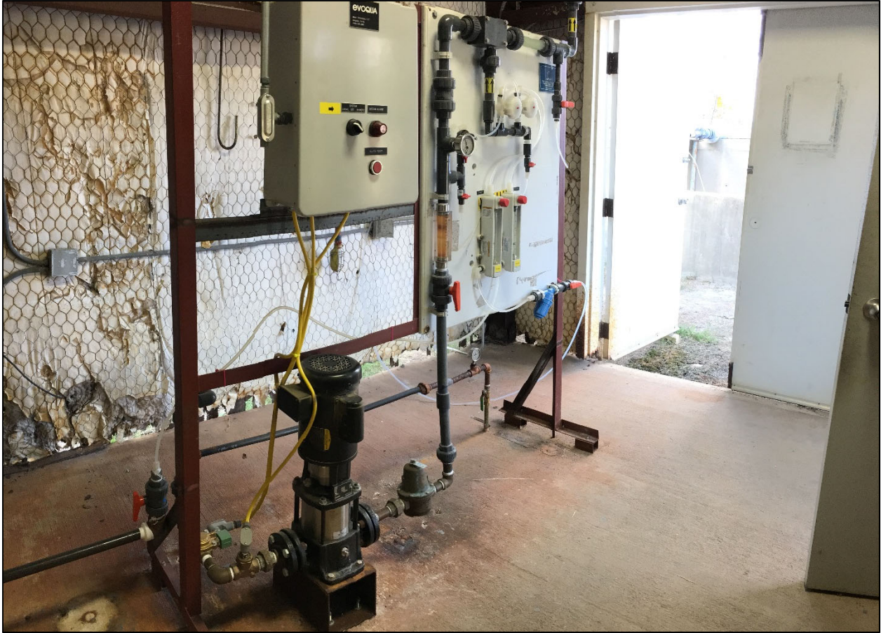
Figure 5-22: New Boston Road WTP Chlorine Dioxide System
