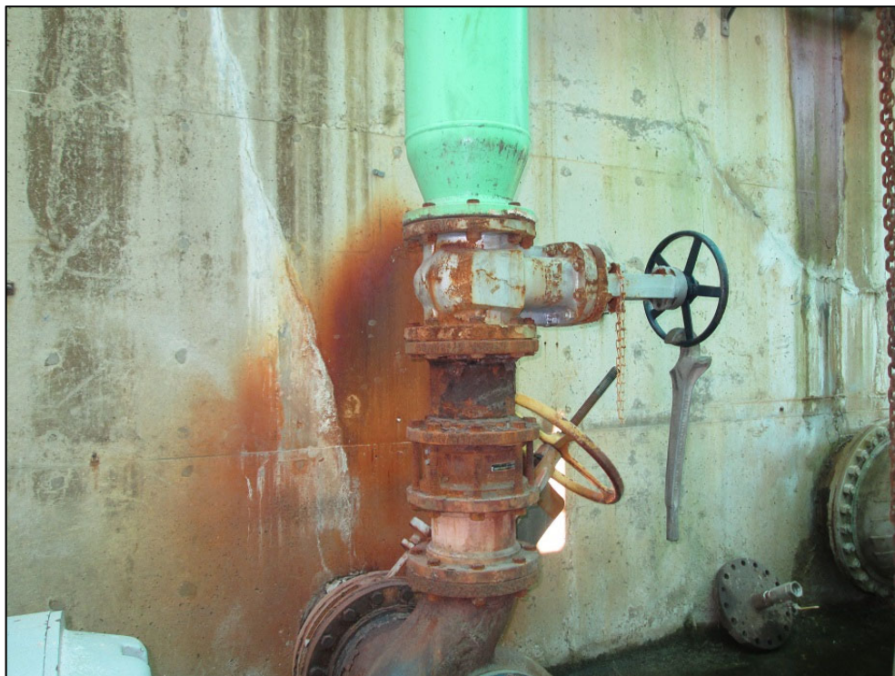
Figure 5-103: Ineffective Coating at GPI WTP Showing Corrosion
