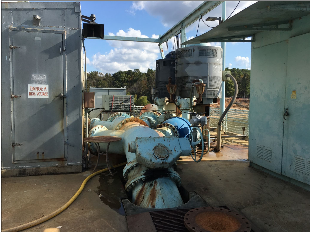
Figure 5-76: GPI WTP Intake Pump Station Pumps and Piping Showing Deficient Coating
