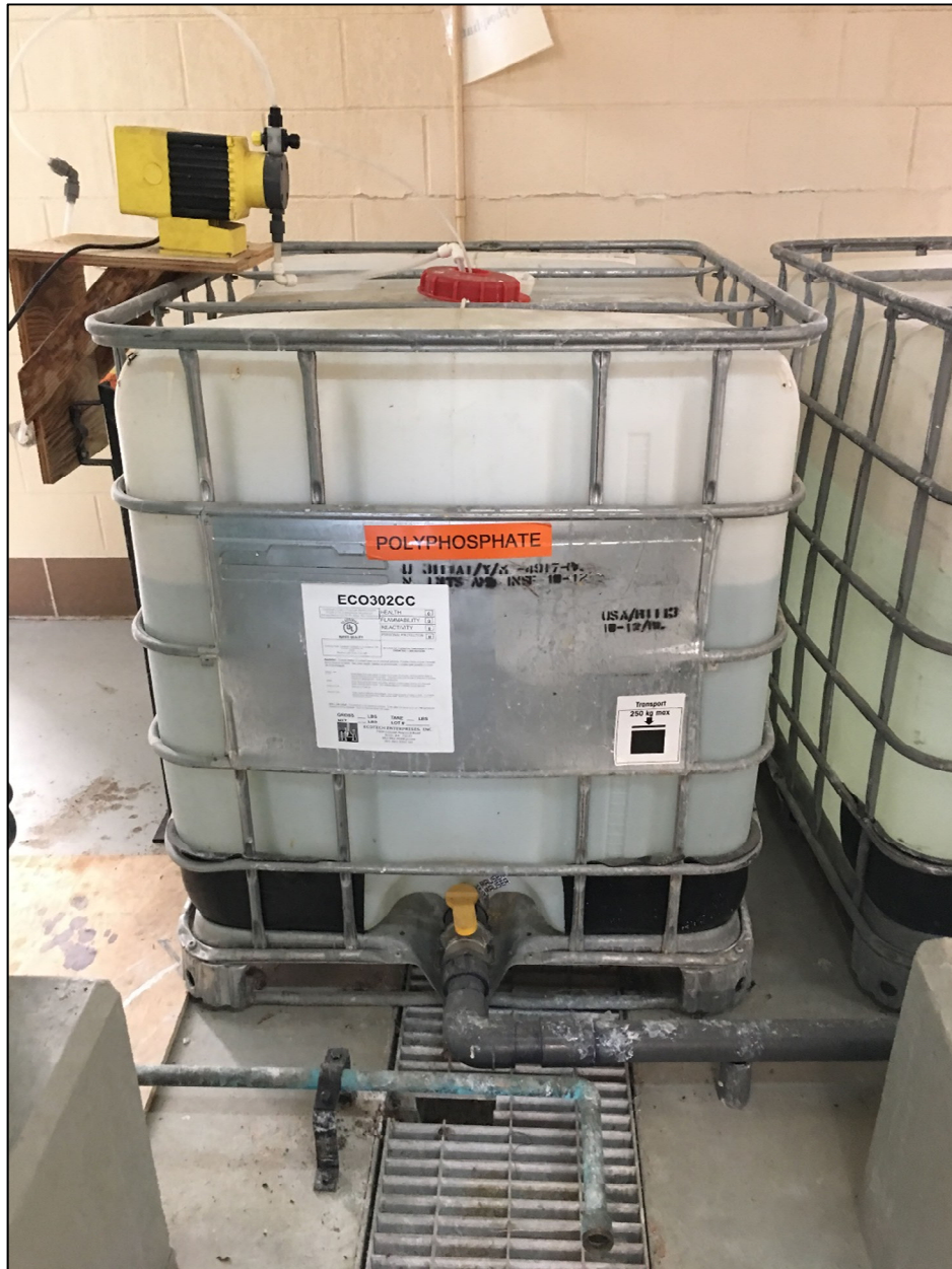
Figure 5-55: Millwood WTP Polyphosphate Feed System
