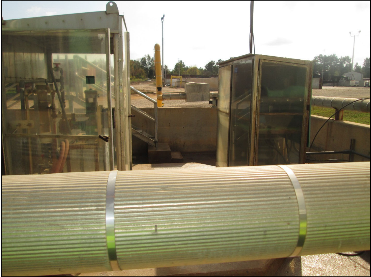
Figure 5-100: GPI WTP Sodium Hypochlorite Feed System Enclosures
