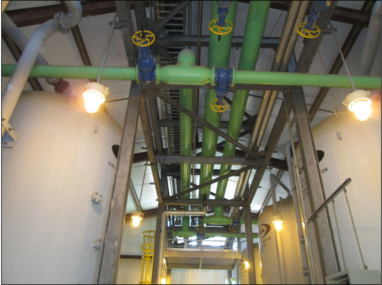
Figure 5-97: GPI WTP GAC Contactor Piping Shown in Good Condition
