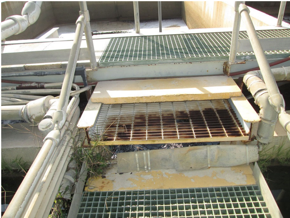
Figure 5-110: Example of Corrosion of Stairs at GPI WTP
