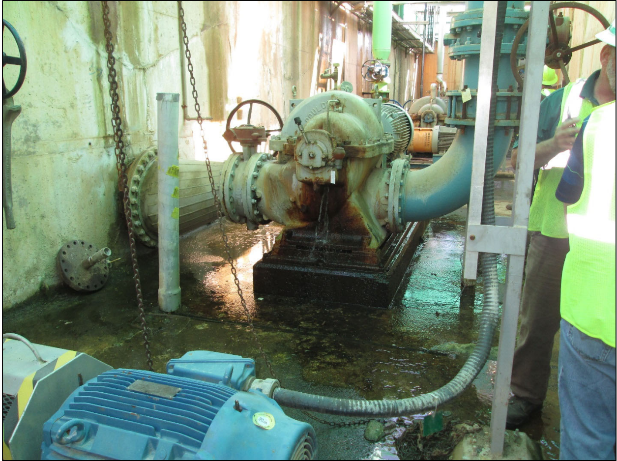
Figure 5-95: GPI WTP Backwash Pump Showing Corrosion
