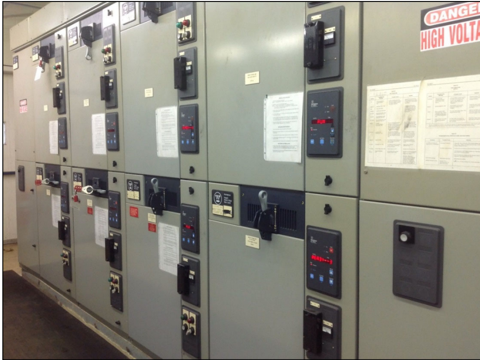
Figure 5-86: Main Switchgear at GPI Intake Recently Replaced
