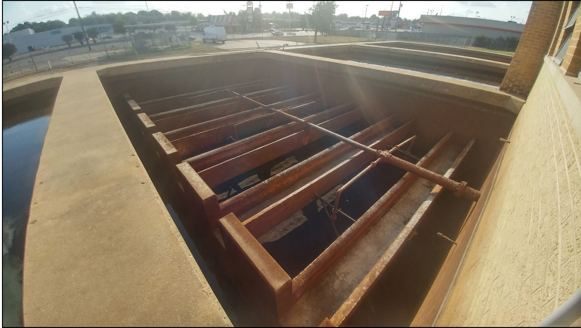
Figure 5-32: Observed Corroding of Metals in Bay at New Boston Road WTP
