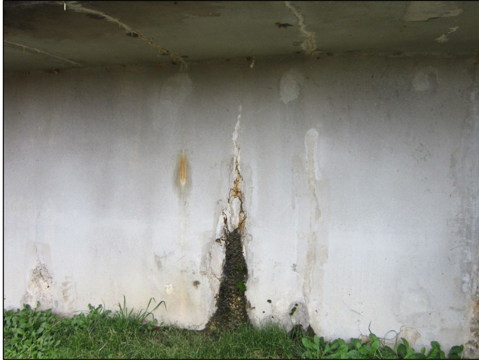
Figure 5-59: Observed Cracking on Wall of Basin at Millwood WTP
