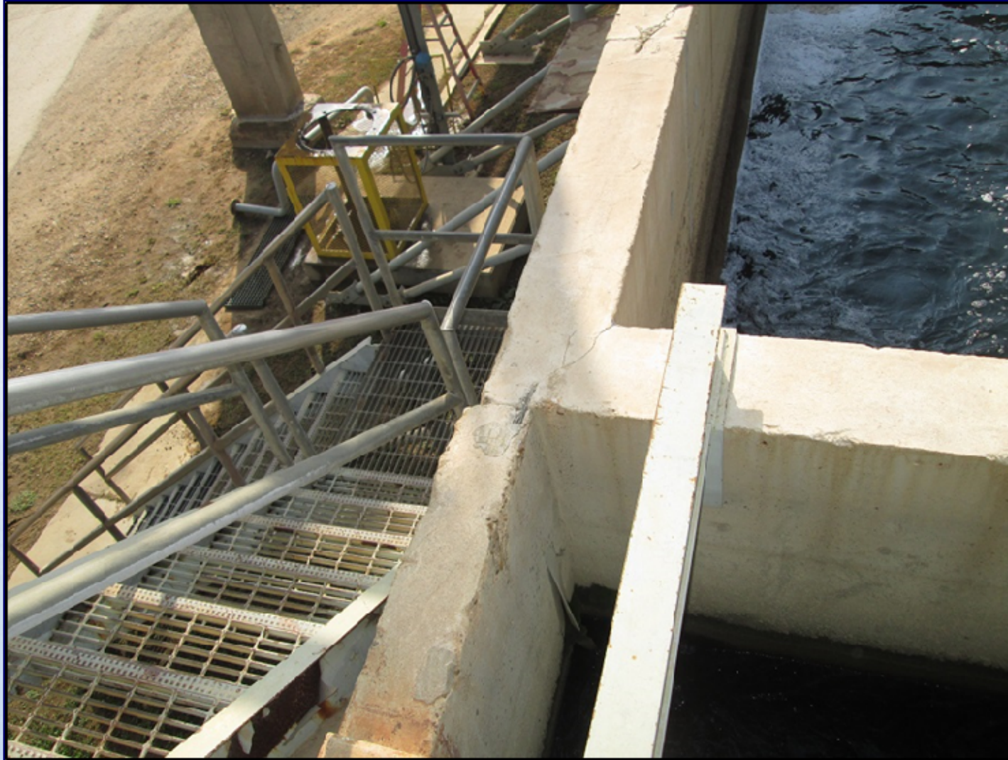
Example of Cracks in Basin Wall at GPI WTP.
