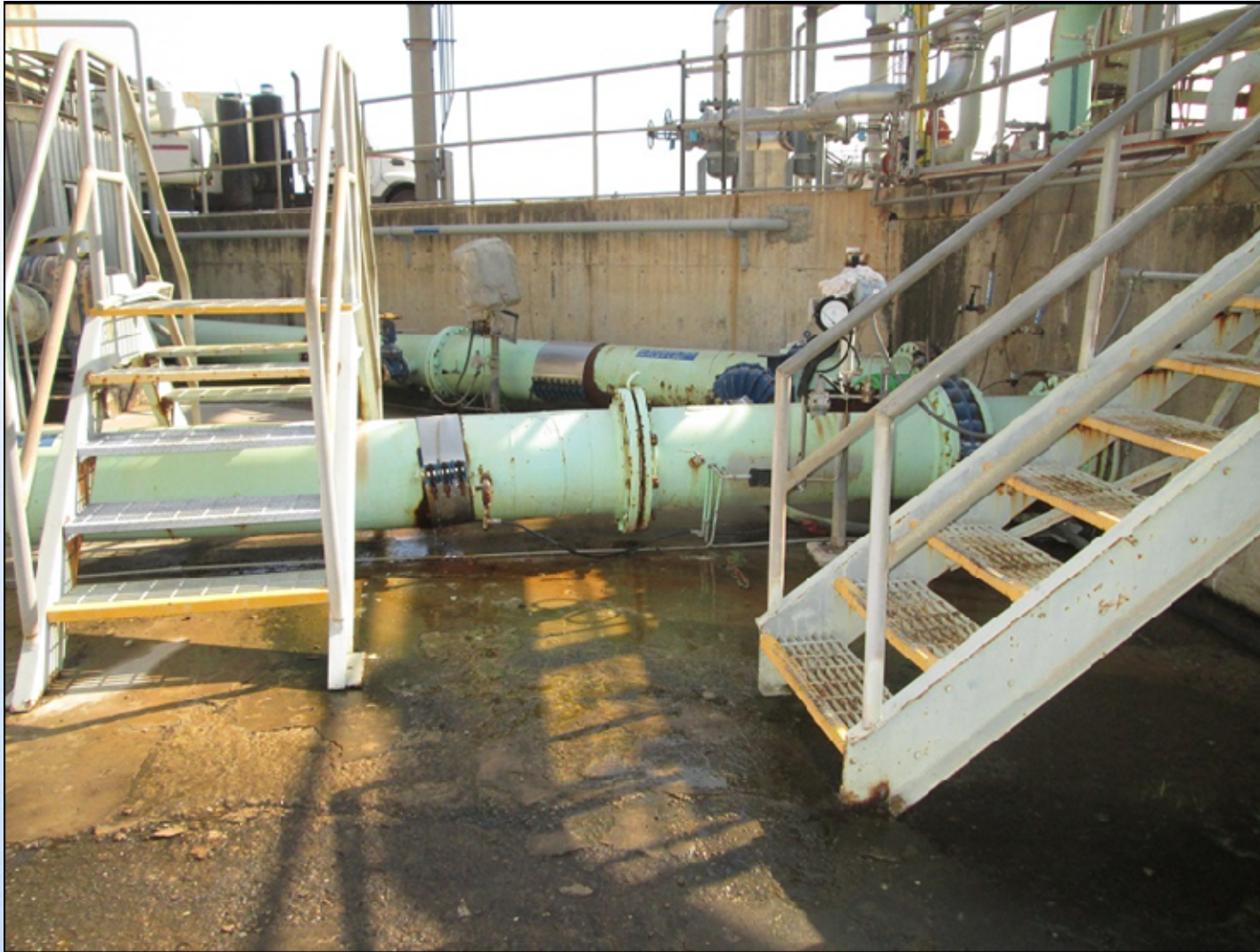
Aged Pipes with Pipe Repair Clamps at GPI WTP Showing Corrosion.
