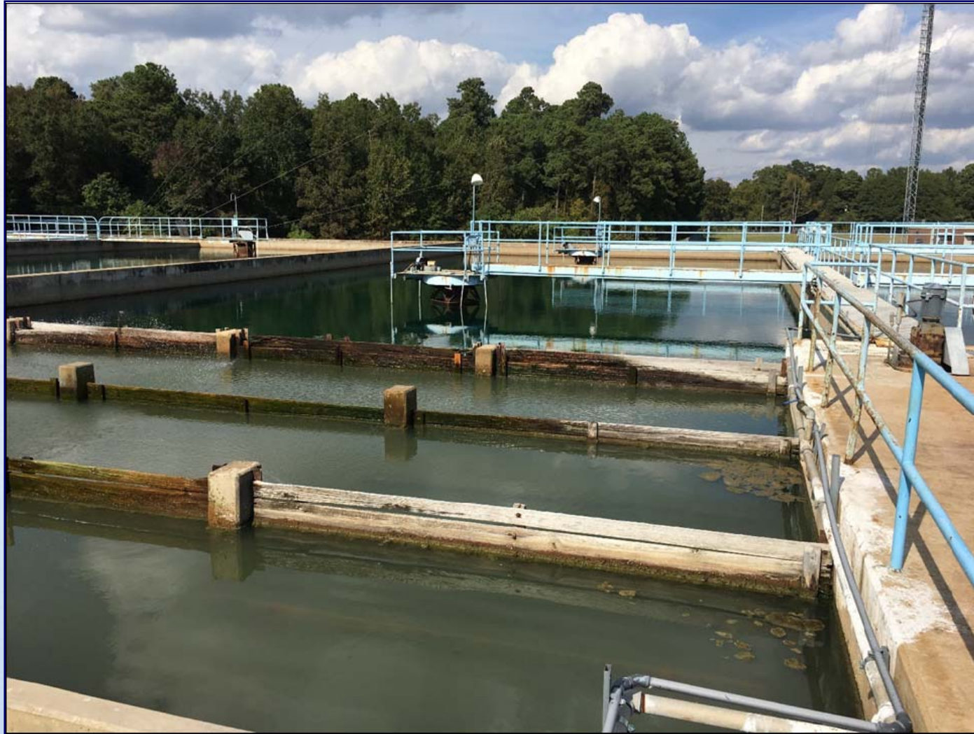
New Boston Road WTP Flocculation/Sedimentation Basins showing baffles and sludge collectors that are past their expected useful life.
